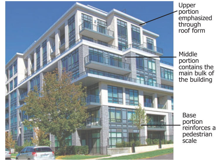
Fig. 6.6.5d - Apartment Buildings should be Designed to Establish Distinct Base, Middle and Upper Portions
