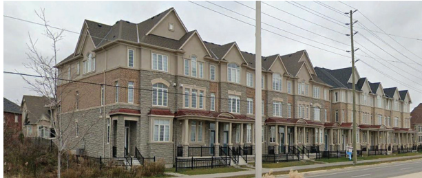
View of Existing Residential on the West Side of Neyagawa Blvd.
