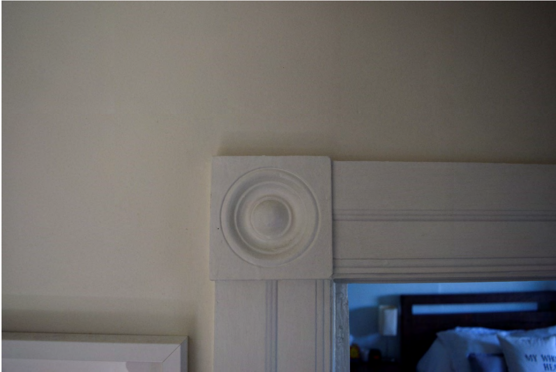
Image 33: Corner blocks on second floor
