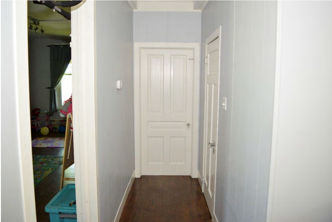
Image 15: Rear 1/4 of c.1911 residence, entrance to first floor washroom is on right, note the use of 4'x8' panelling as wall finish, non-original
