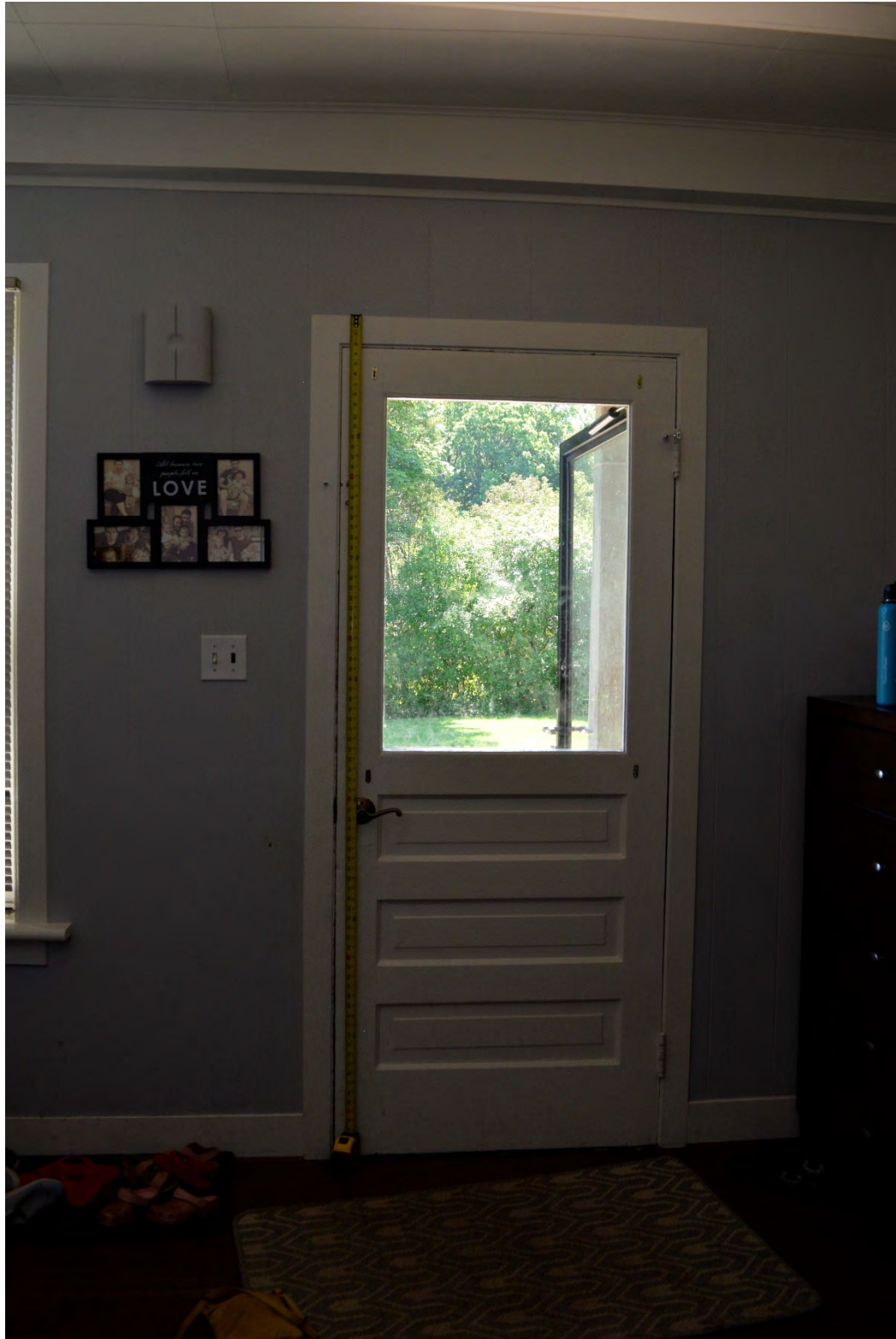
Image 22: Original frame and panel wood door on south face of residence, note non-original trim and baseboard
