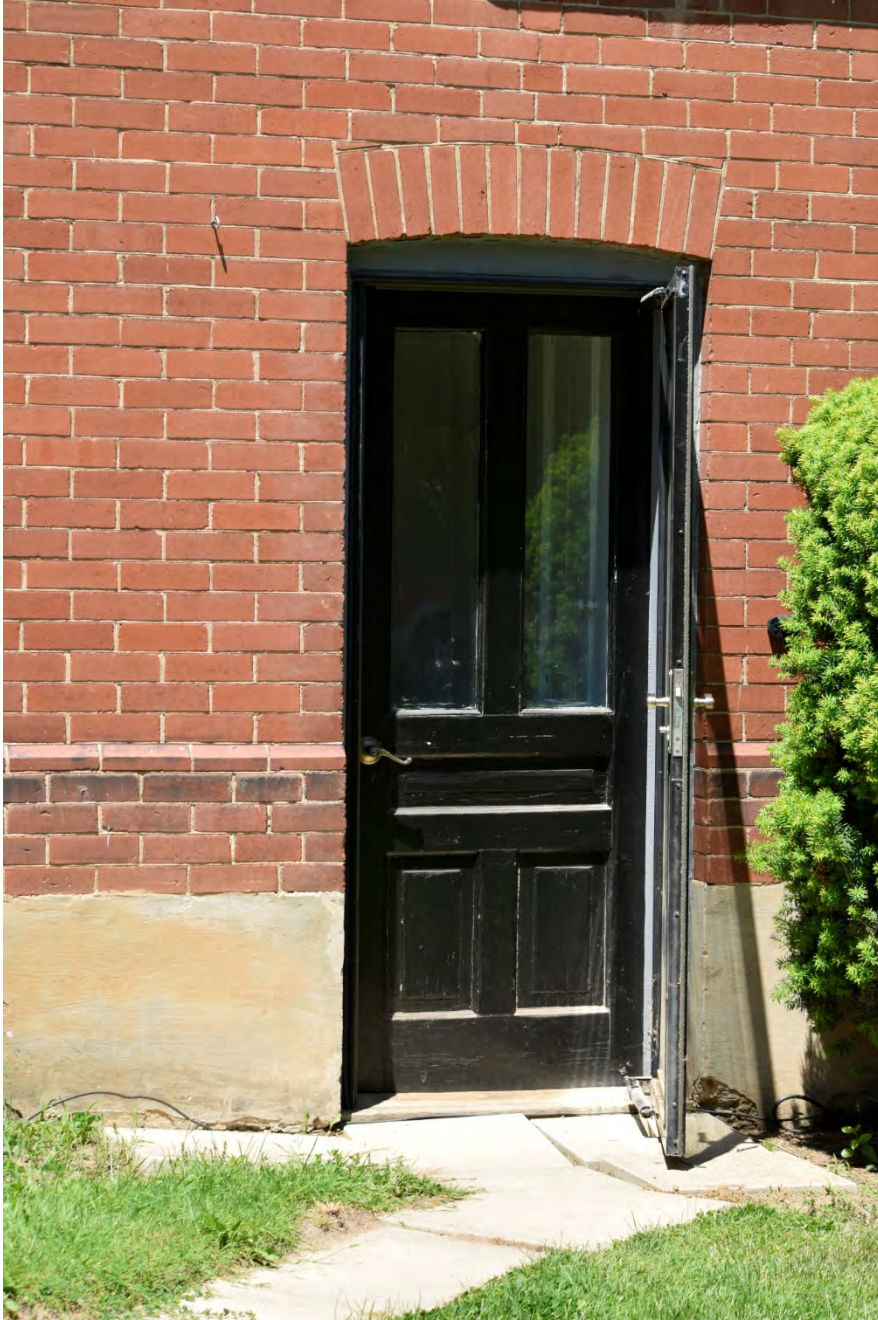
Image 10: Original frame and panel door with glass on south face, note jack arch and 45° beveled brick plinth cap
