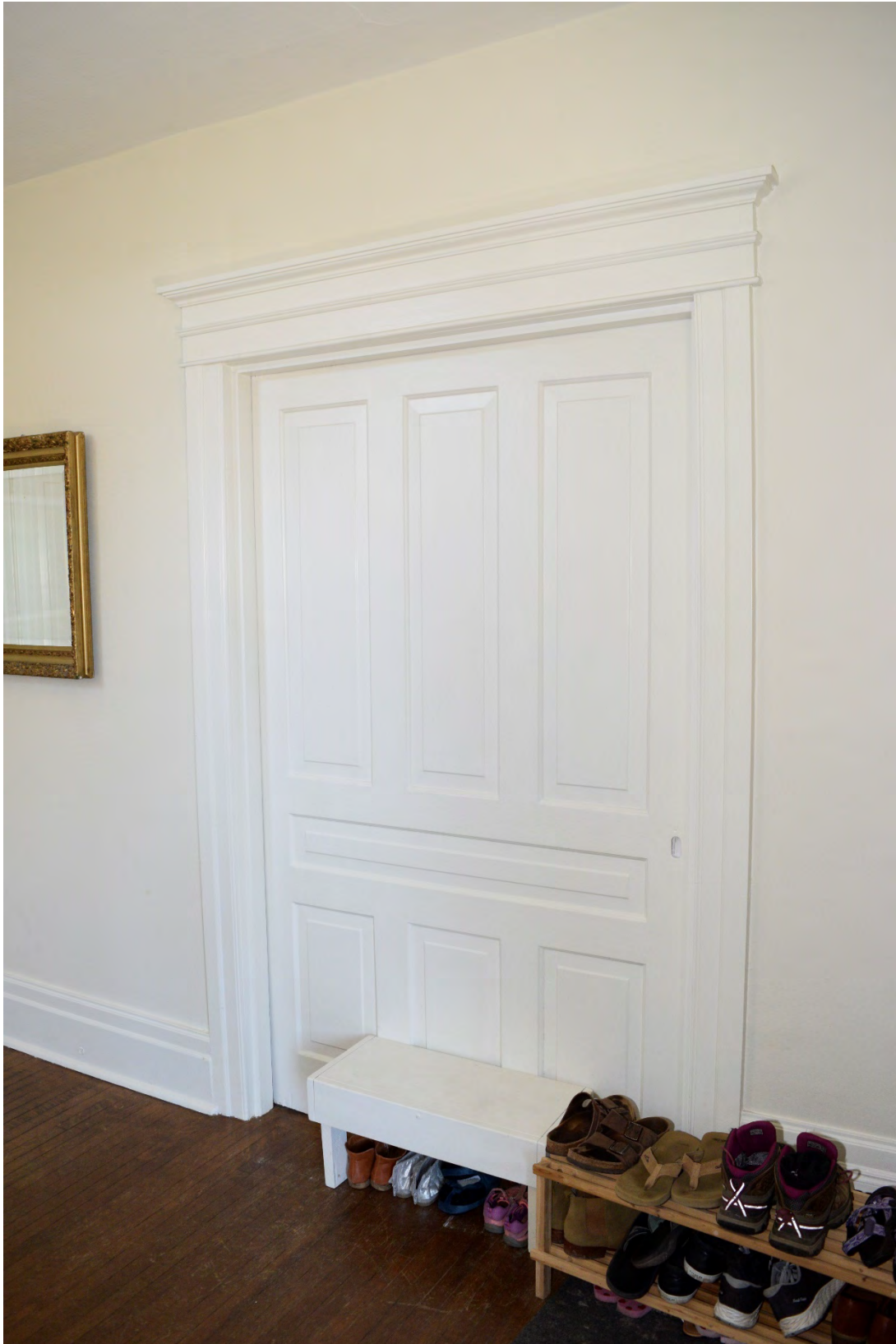
Image 32: Representative example of original woodwork on first floor including pocket door, cabinet head trim and baseboard
