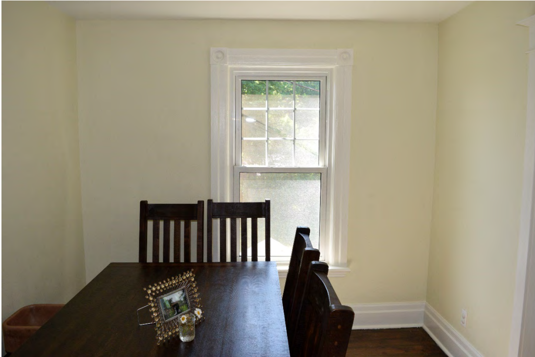
Image 28: Second floor dining room in c.1911 residence, note use of corner blocs at window trim
