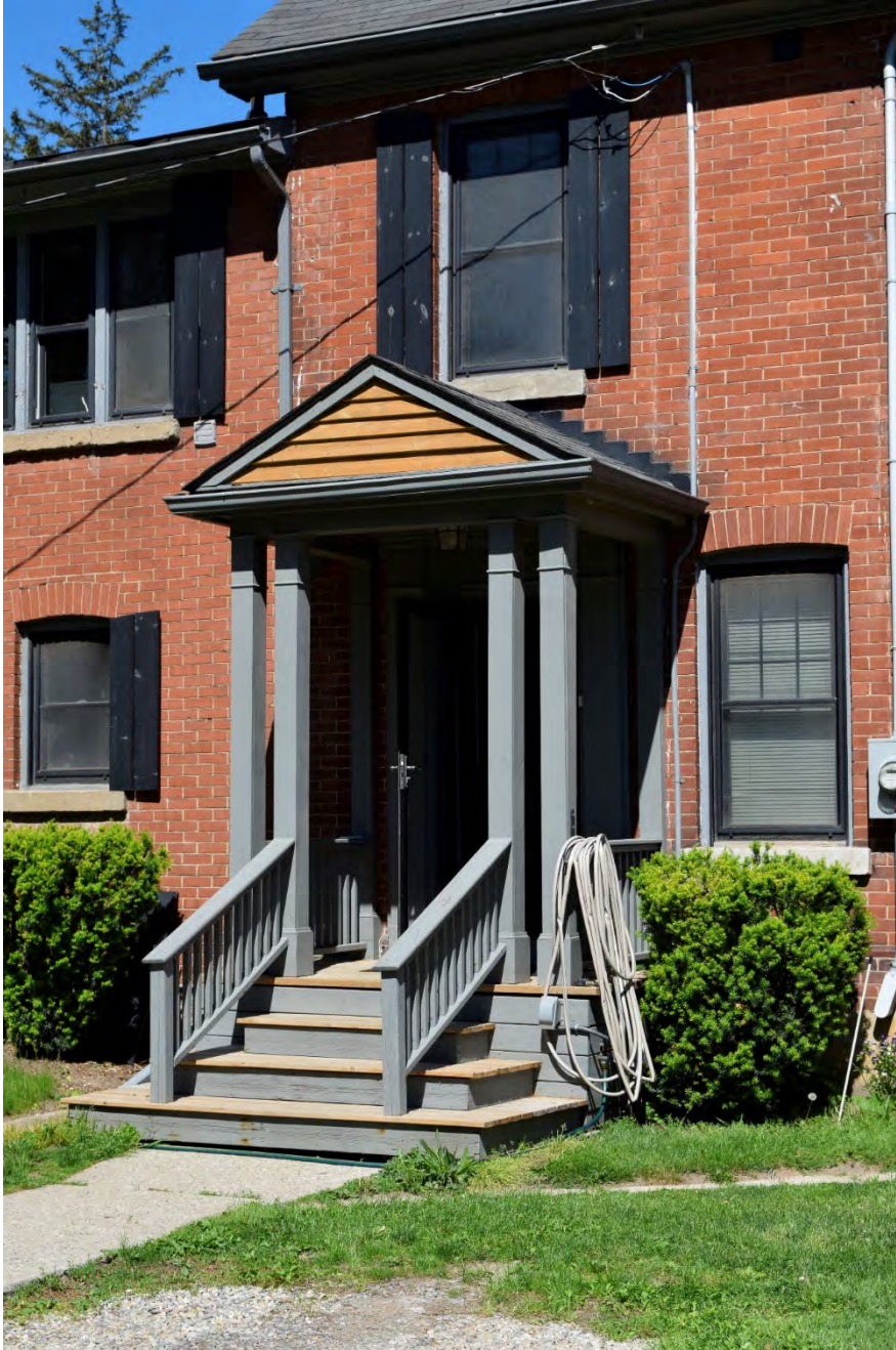
Image 12: Porch on south face of residence, only gable roof structure appears original
