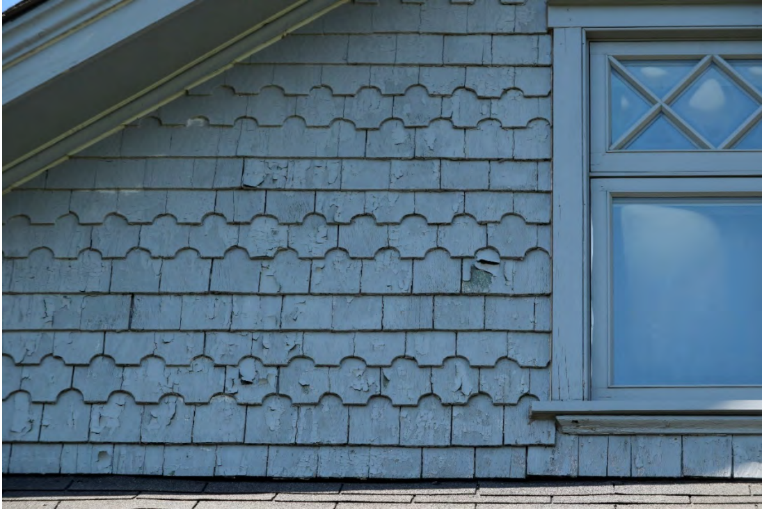
Image 7: Decorative cedar shakes used in gable ends, note condensation on windows indicating broken seals in need of replacement
