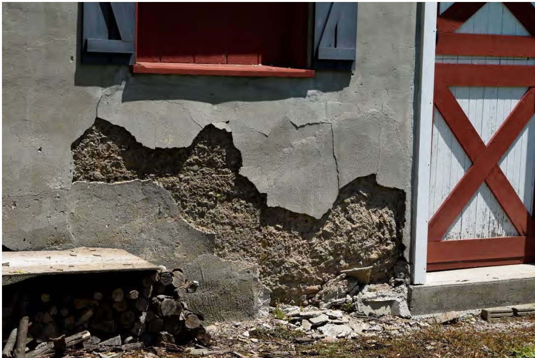
Image 43: Parge coat failing revealing coarse concrete foundation, note new concrete step associated with door
