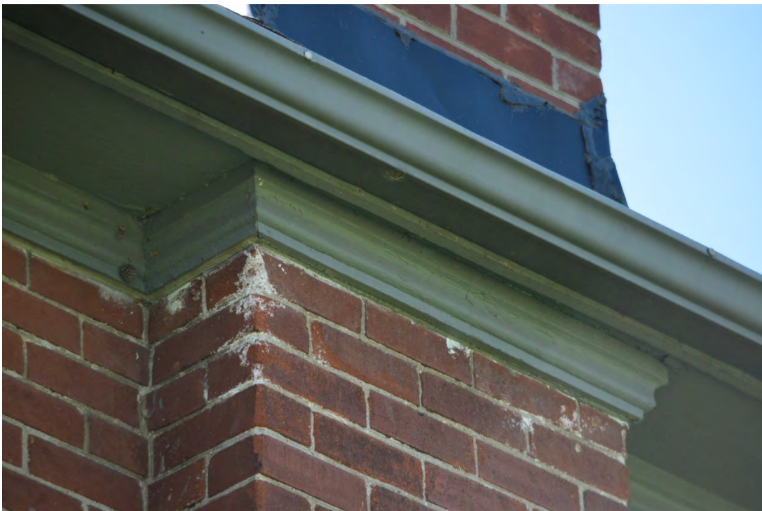
Image 8: Typical moulded freeze under eaves
