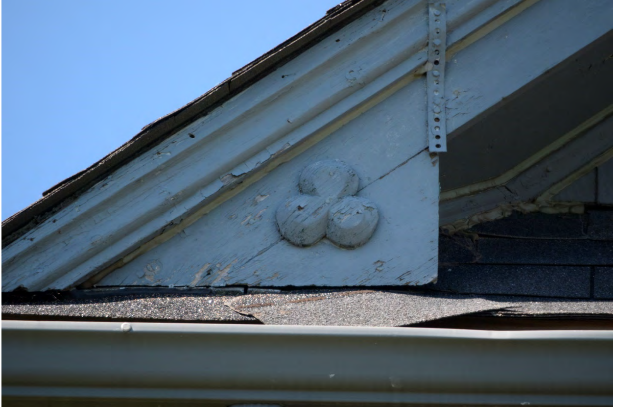
Image 9: Decorative trefoil detail on closed pedimented gable end, signs of water infiltration and evidence of attempted repair
