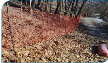
Tree protection fencing to be installed
