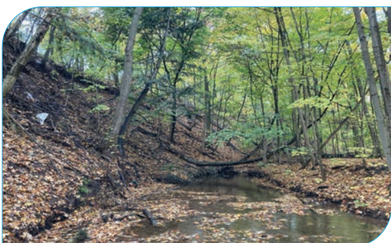
Site: E19 Score: 44 Issue: Valley wall contact along meander bend (90 degrees); gabion basket protection in fair condition (leaning) Risk: Pedestrian trail system; private property Length: 20 – 50 m
