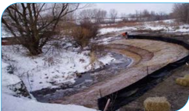
Temporary silt fencing for erosion and sediment control to be installed
