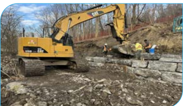
Heavy machinery will be required to build armoured stone structures
