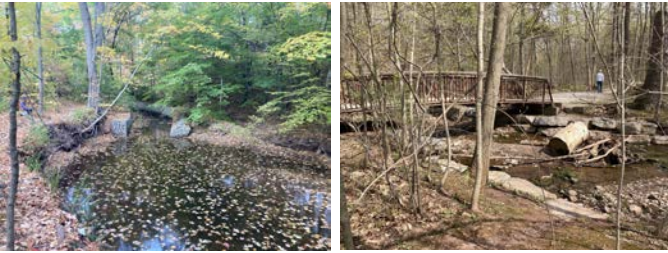
E5: Failing gabion baskets with downstream scour pool. Risk to pedestrian bridge/trail
