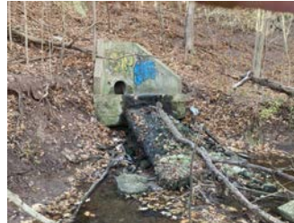
E6: Perched outfall on valley slope with suspended drop structure and scour pool. Risk to outfall and private properties at top of slope.
