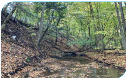
Site: E19 Score: 44 Issue: Valley wall contact along meander bend (90 degrees); gabion basket protection in fair condition (leaning) Risk: Pedestrian trail system; private property Length: 20 – 50 m
