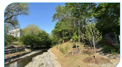
Erosion control blankets to be installed on restored banks
