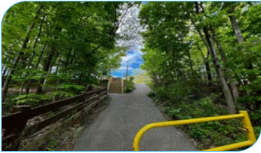
Construction access into creek corridor along existing trail. Tree removals will be required (estimated 100 trees).
