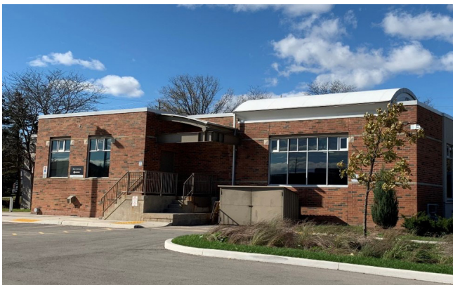
Figure 8: Oakville Public Library, Woodside Branch. One-storey building directly adjacent to subject site with pedestrian linkages. Source: Fotenn Site Visit
