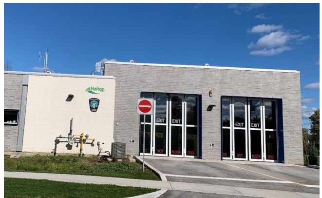
Figure 9: EMS Station. One-storey building adjacent to subject site and south of public library. Source: Fotenn Site Visit
