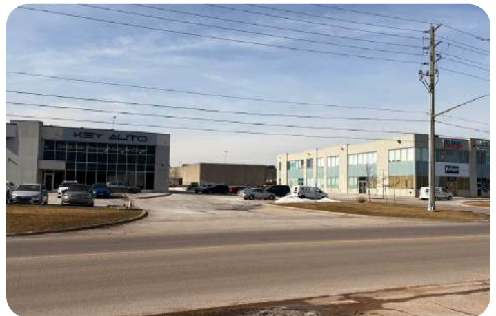
Commercial and office buildings at 2195 Wyecroft Road
