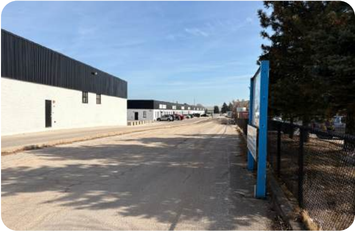
Subject site looking east from the western entrance driveway
