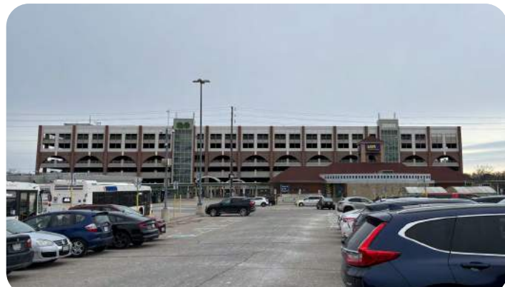
Oakville GO Bus parking structure
