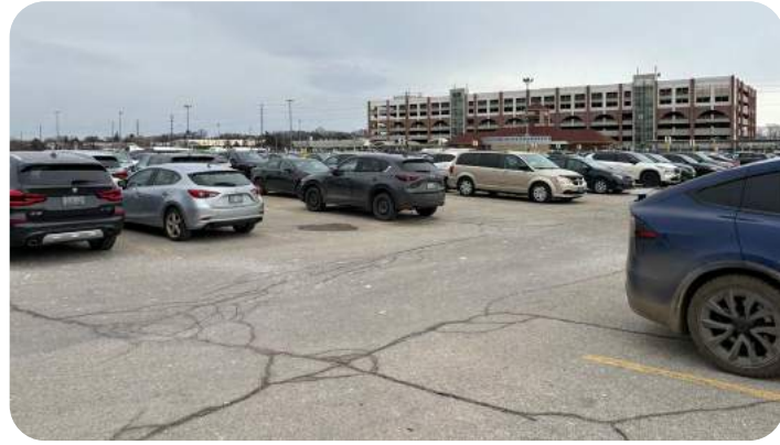
Oakville GO Station parking lots
