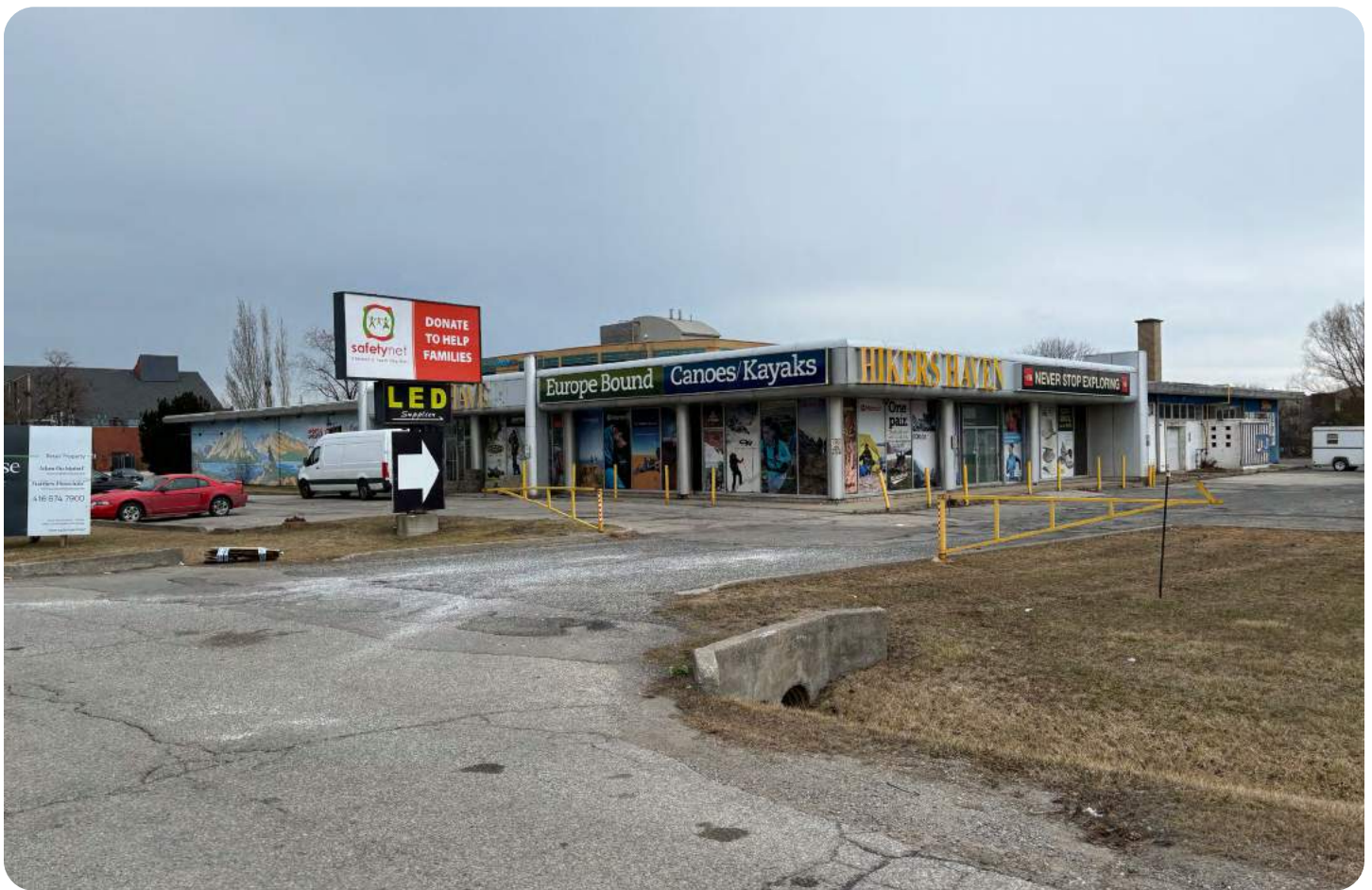
166 South Service Road
