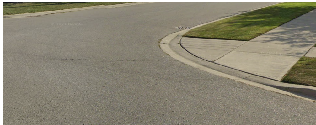
Example of existing barrier-free curb ramp in adjacent neighbourhood.
