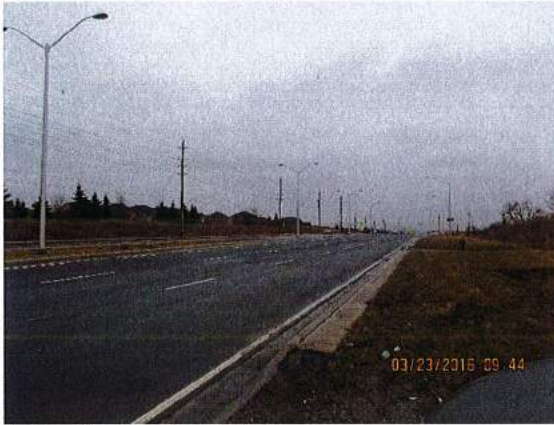
7. Dundas Street East; facing west
