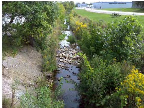
Photo 22: Downstream view of channel from Wycroft Road on September 7, 2018.
