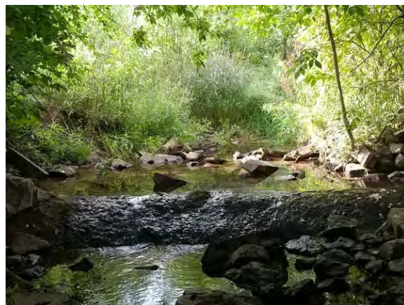
Photo 23: Channel reach upstream of the QEW showing instream barrier (September 7, 2018).
