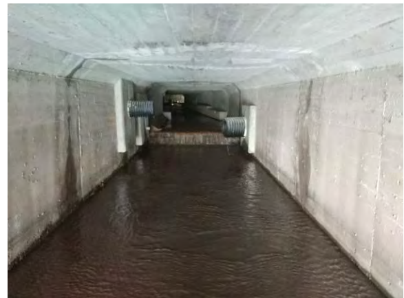
Photo 18: Inside culvert, upstream view of perch.
