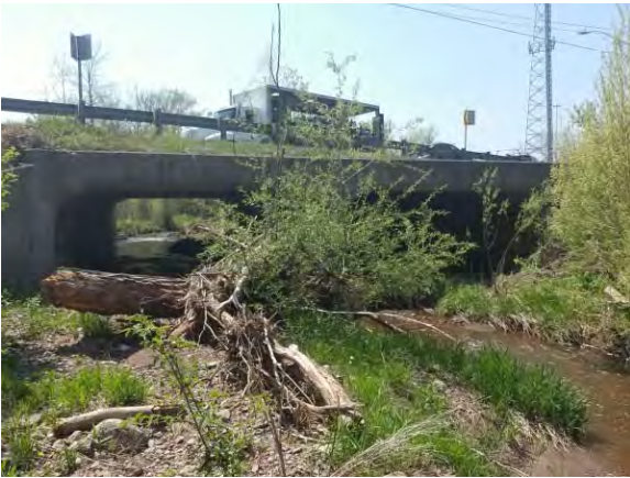
Photo 7: Upstream view of the structure outlet, showing large log and dry vegetated point bar.
