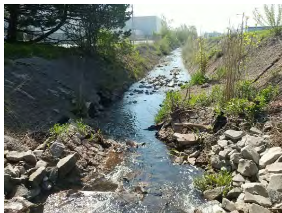
Photo 17: Another downstream view from culvert, showing rip rap and concrete sections instream.
