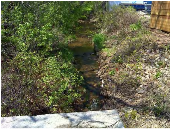
Photo 30: Upstream view of channel from the top of the culvert.
