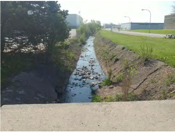
Photo 13: Downstream view of McCraney Creek (May 17, 2018).
