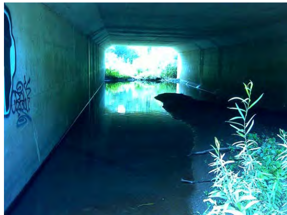
Photo 12: Upstream view of north structure cell (September 7, 2018).
