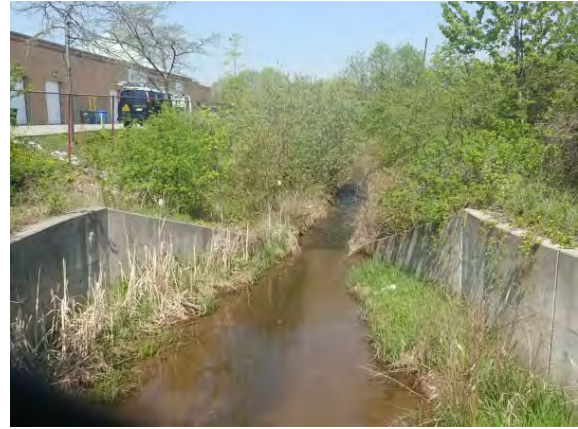
Photo 25: Upstream view of creek showing widened inlet area.
