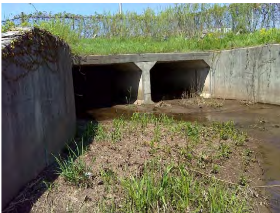
Photo 28: Upstream view of culvert outlet.
