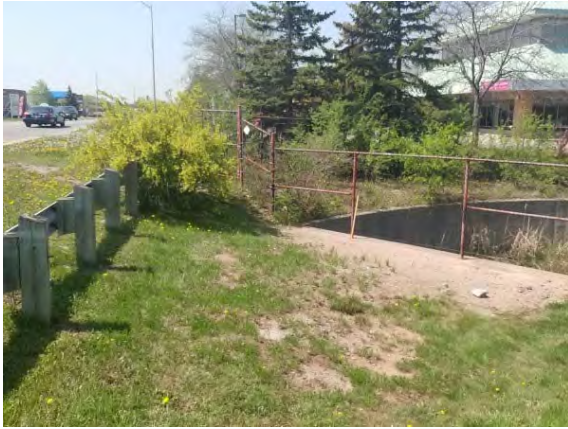
Photo 24: Westerly view of culvert inlet and distance from Wycroft Road.
