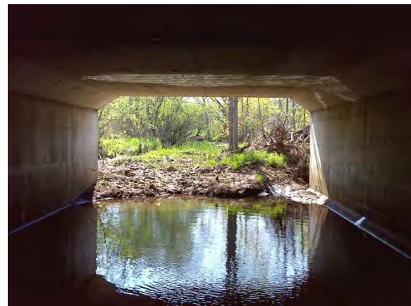
Photo 6: View of backwater within the north structure cell.
