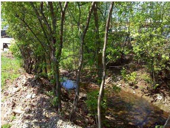
Photo 32: Upstream view of channel showing narrow riparian and soil dumping along the west bank.
