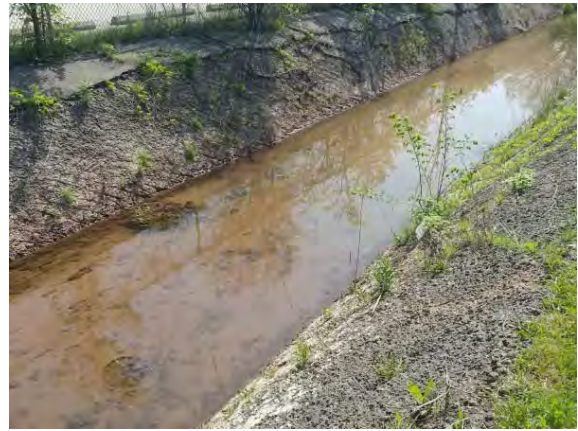
Photo 20: Flat morphology and soft substrate deposition area, near the downstream edge of the assessment area.
