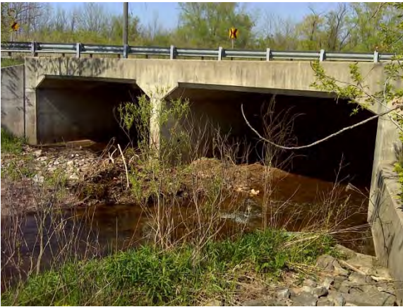
Photo 1: Structure inlet, view from southwest bank (May 17/2018).
