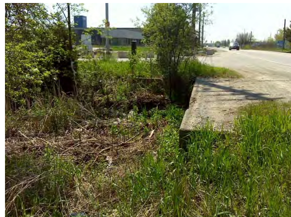
Photo 35: Westerly view of culvert outlet and vicinity.
