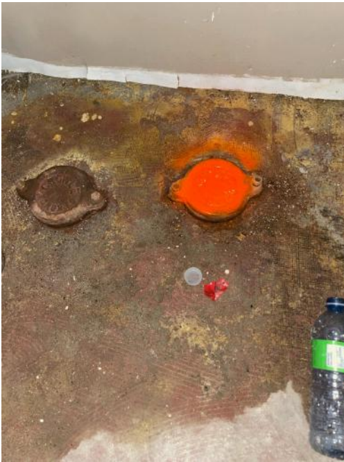
View of sanitary cleanout in basement (storm left), looking south (towards Robinson).
