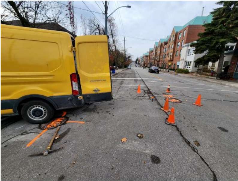
View of EX-STM & EX-SAN-1, looking west.
