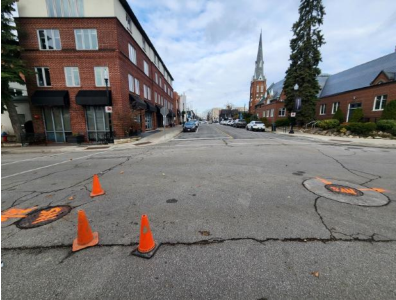
View of EX-SAN-1 & EX-SAN, looking north.
