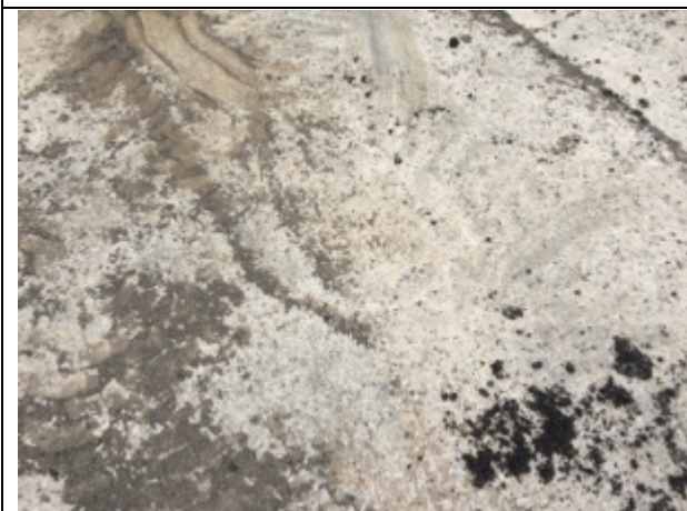
Image 17 Concrete Ground Conditions
