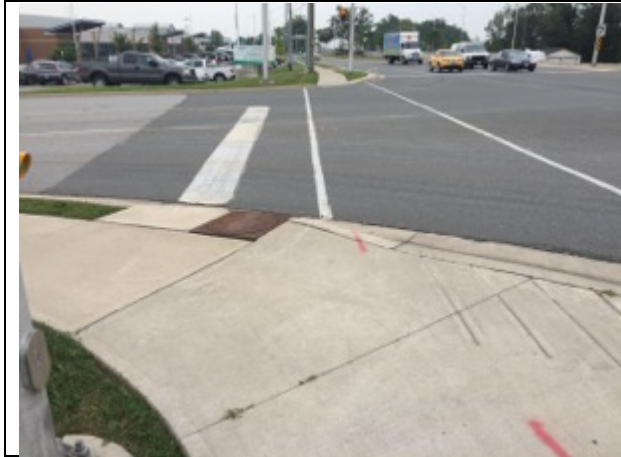
Image 9 Assessment Conditions: Lawn area, Concrete sidewalk, Asphalt roadway, Asphalt parking lot
