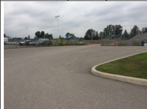
Image 5 Asphalt parking lot
