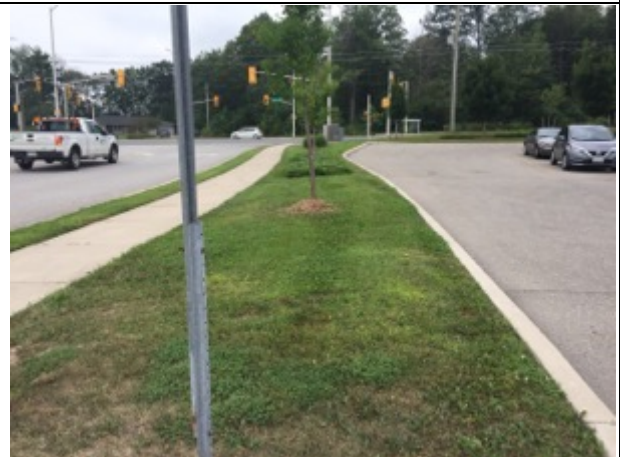
Image 6 Assessment Conditions: Lawn area, Concrete sidewalk, Asphalt roadway, Asphalt parking lot
