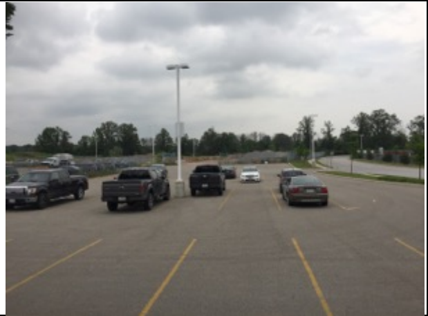
Image 10 Asphalt Parking lot
