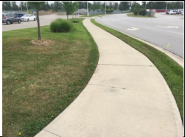
Image 8 Assessment Conditions: Lawn area, Concrete sidewalk, Asphalt roadway, Asphalt parking lot
