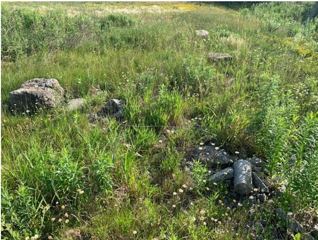
Photograph No. 6– View of the concrete debris in the southern portion of the Site and the location of borehole BH105-21.
