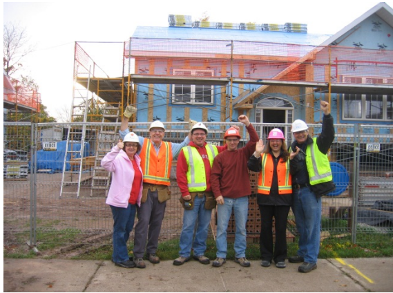
Holcim Volunteers at Oakville Habitat for Humanity Build
