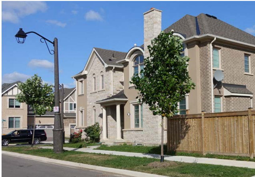
Fig. 6.4.1 - Image example of a corner lot dwelling in North Oakville that addresses both street frontages with the long elevation facing the flanking street
