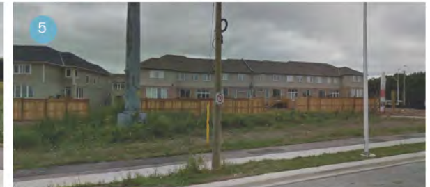
Existing townhouses with reverse frontage on Upper Middle Rd.
