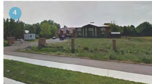
Existing dwelling on Bronte Road
