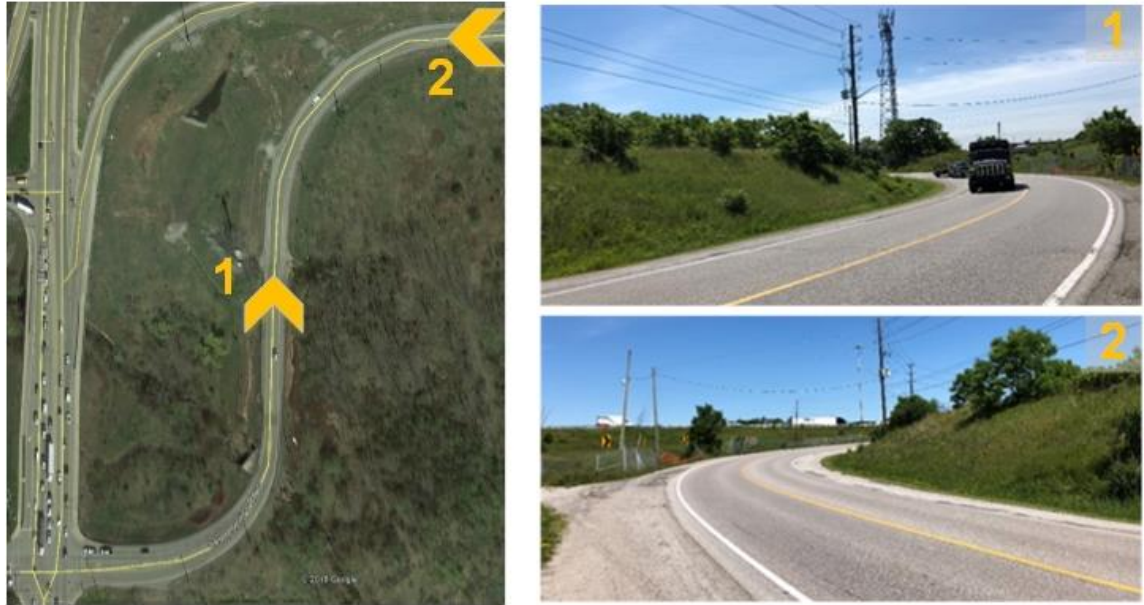
Exhibit 3-17: Reverse Curve on South Service Road
