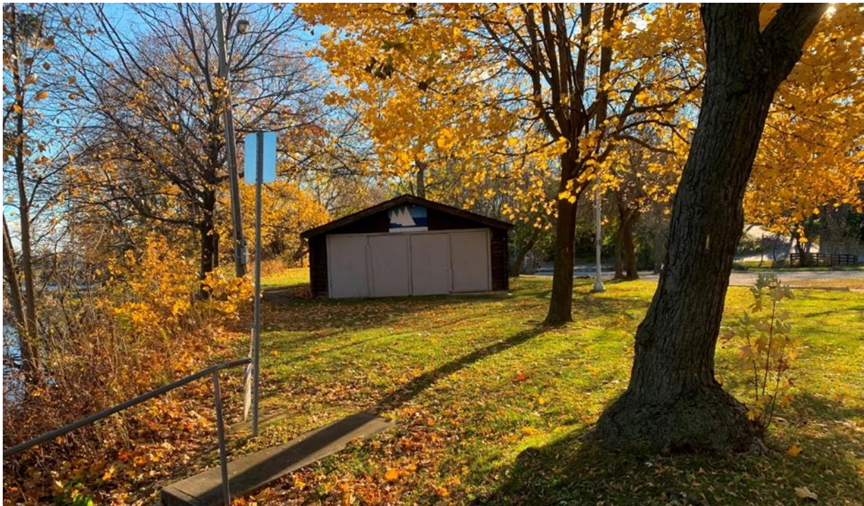
Photo 3.6: Top of Bank at Berta Point
