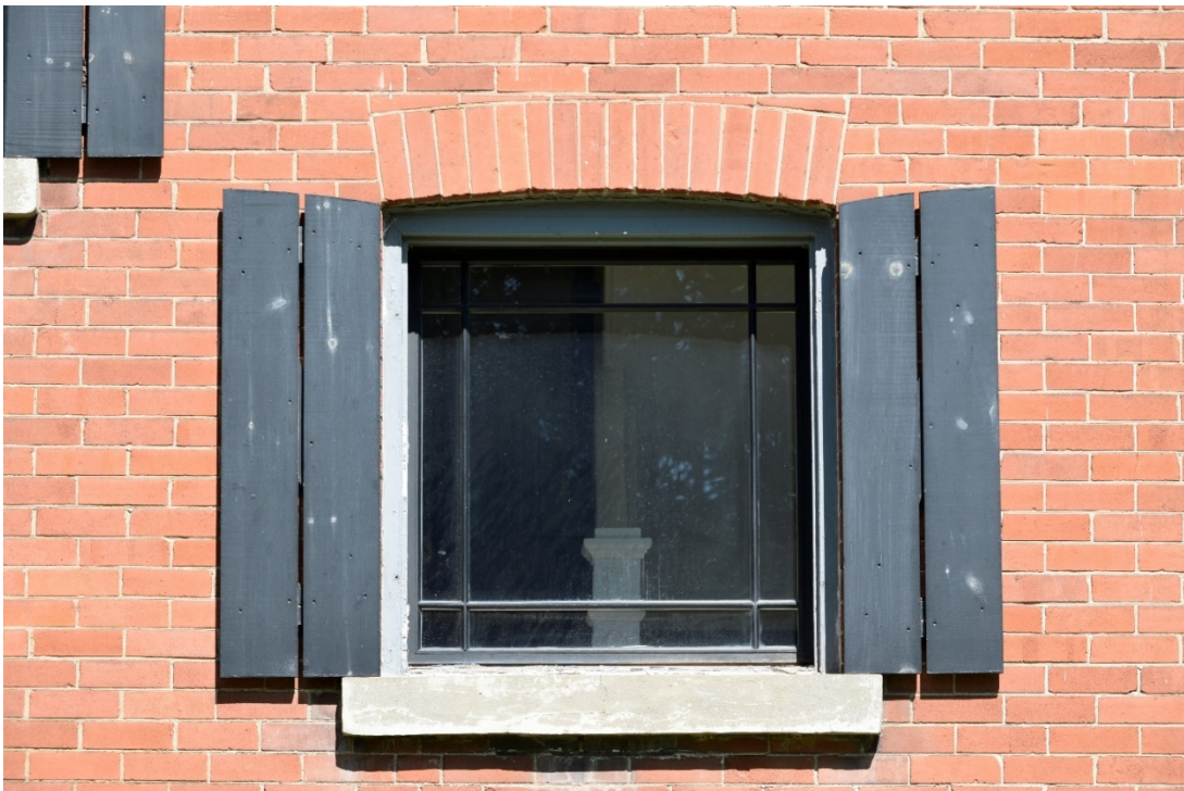
Image 6: Typical window with jack arch and cast lug sill, window and shutters are non-original
