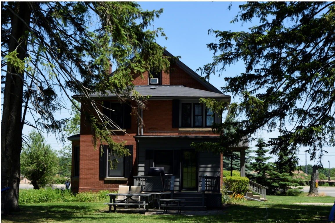
Image 4: West facade of residence, note truncated hip roof of c. 1920 addition, facing east
