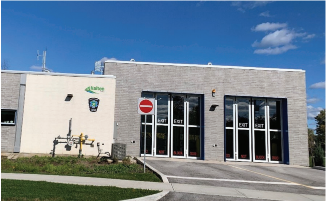
Figure 9: EMS Station. One-storey building adjacent to subject site and south of public library. Source: Fotenn Site Visit
