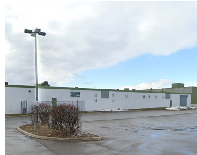
Figure 15. Looking west towards 201 Speers Road heritage building
