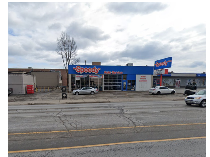
Figure 18. View of low-rise commercial buildings located south of the subject site
