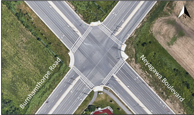
Figure 3: Intersection of Neyagawa Boulevard at Burnhamthorpe Road
