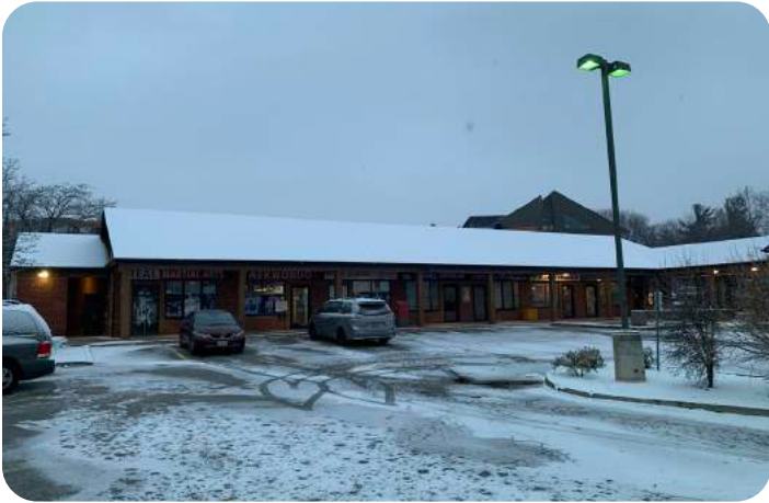
Subject Site, 2163 Sixth Line, Northern Portion of the Building
