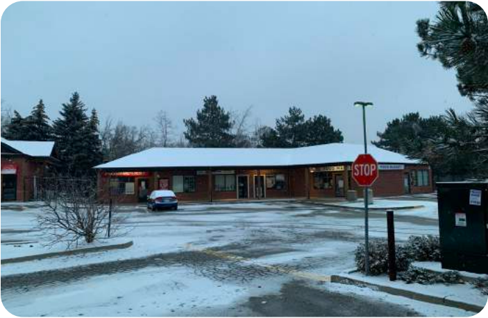
Subject Site, 2163 Sixth Line, Southern Portion of the Building
