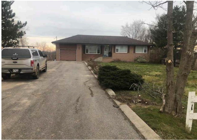
Plate 3 Shows area of tarmac driveway and existing standing structure.
