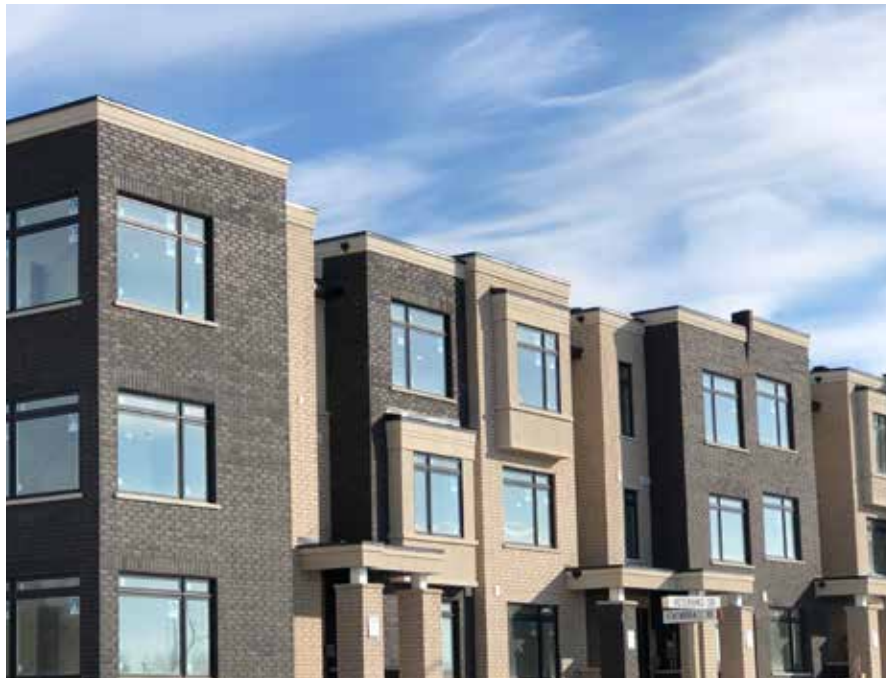
Contemporary roof design
