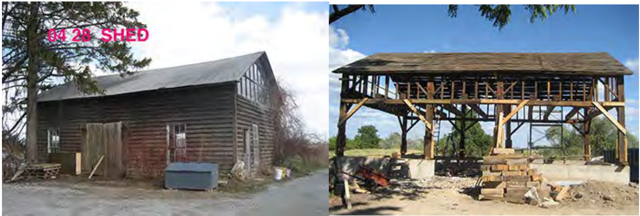
Figure 32: Photo of the original shed (left) and images of it when it was stripped down to the structural timber frame (right). Note the new concrete foundation was added. (Sybil Rampen personal photographs).
