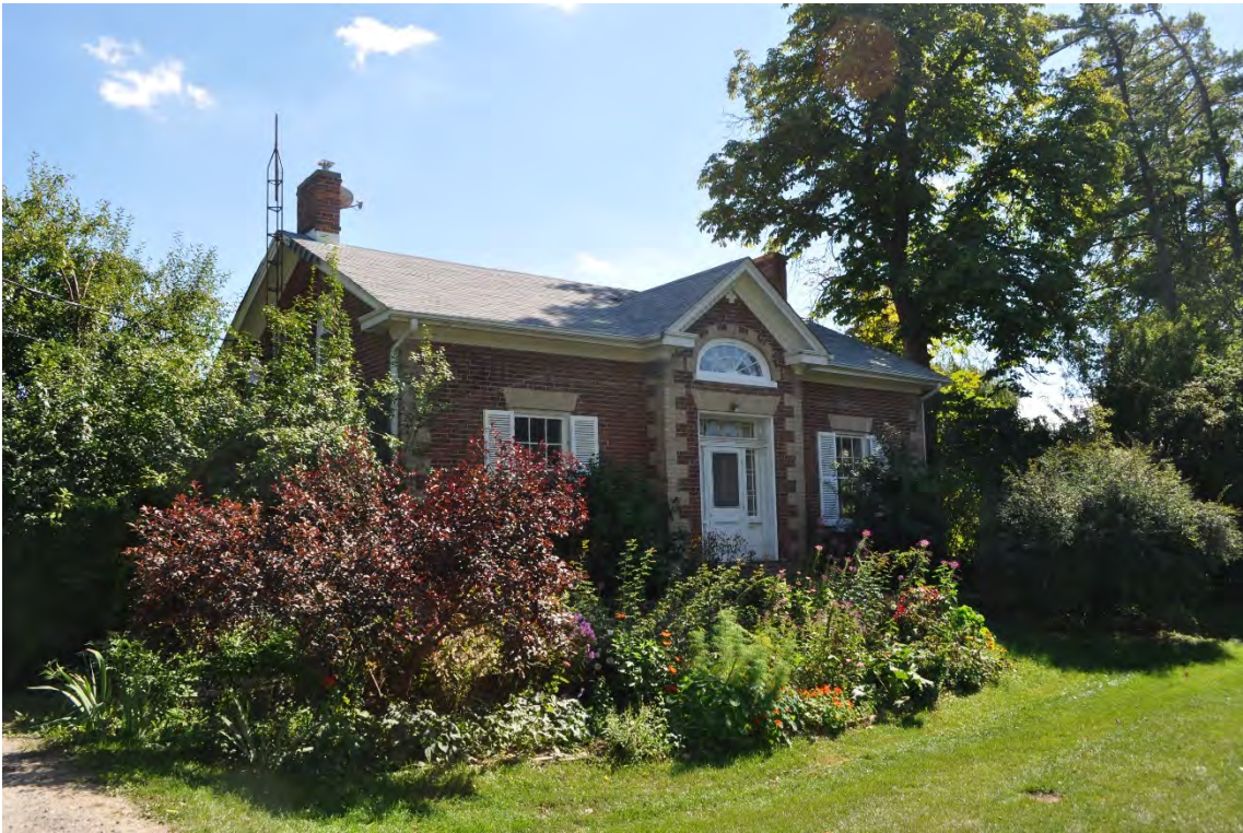
Figure 8: Façade of farmhouse at 1086 Burnhamthorpe Road East (CU 2016).
