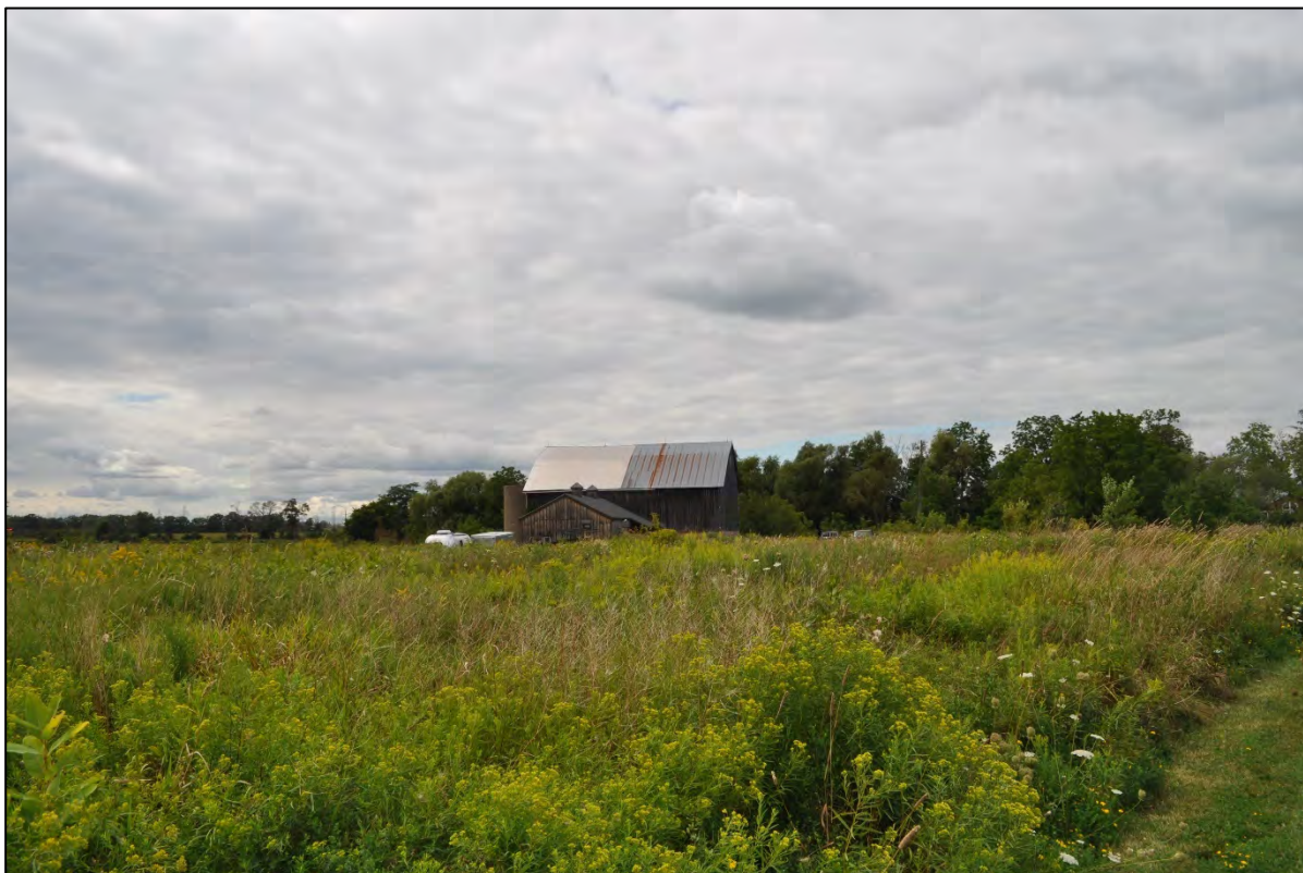
Figure 3: Bank Barn at 1086 Burnhamthorpe Road East, viewed from the labyrinth (CU 2015).
