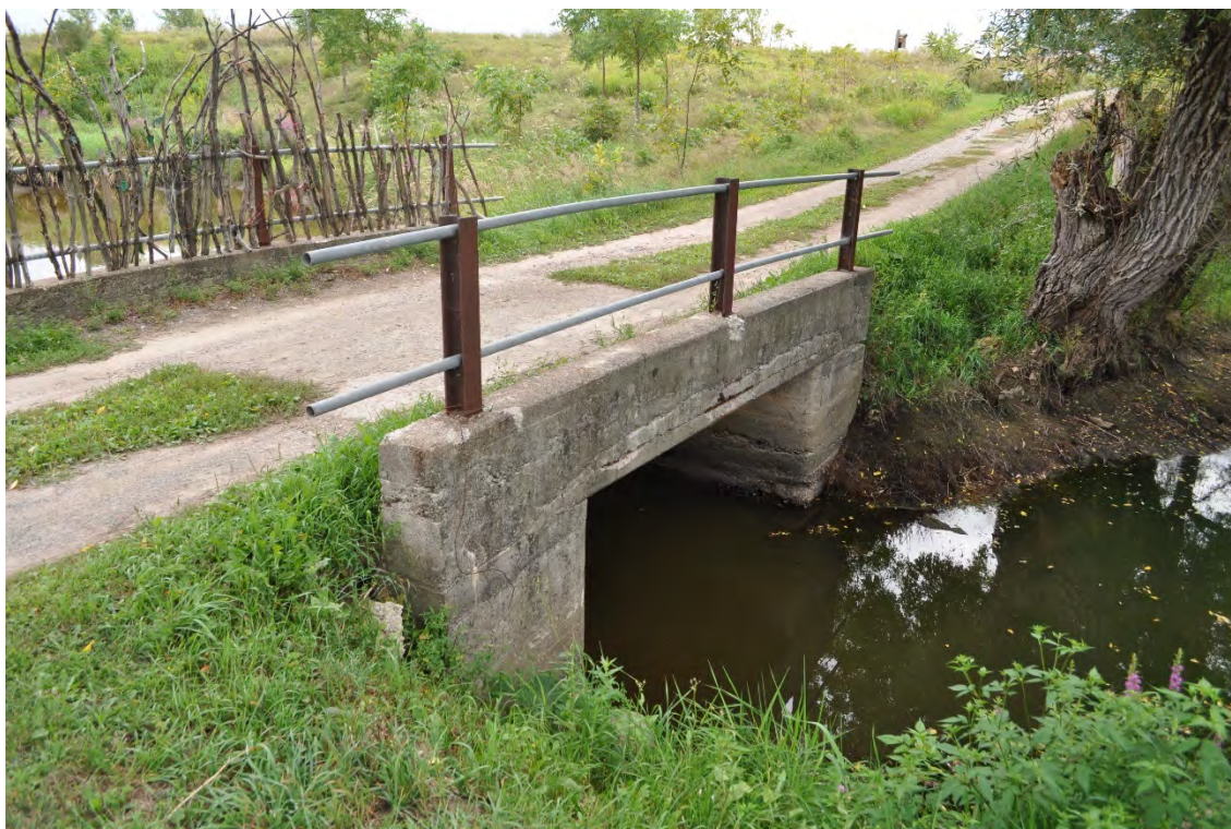
Figure 18: Concrete bridge over Joshua Creek, built circa 1914 (CU 2015).
