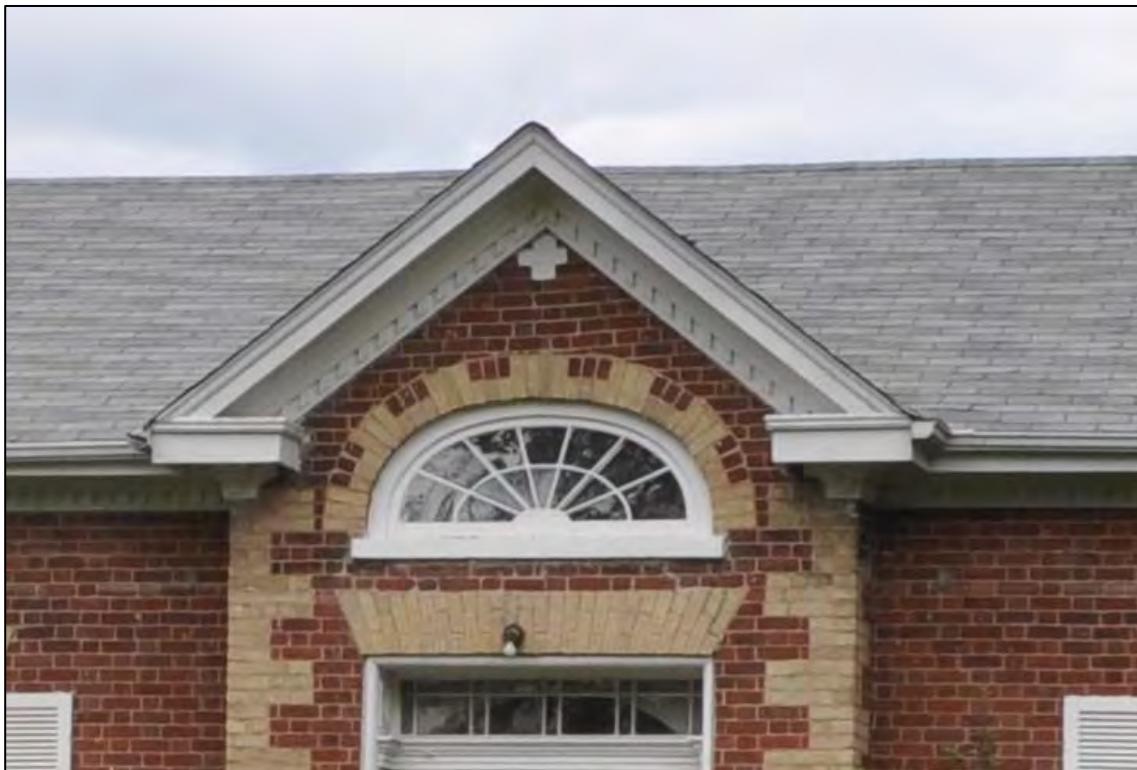
Figure 9: Detail of gable peak (CU 2015).
