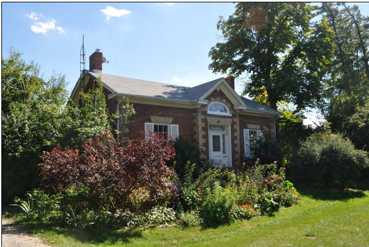
Figure 2: View of façade of the 1853 dichromatic brick farmhouse at 1086 Burnhamthorpe Road East (AB, 2016).
