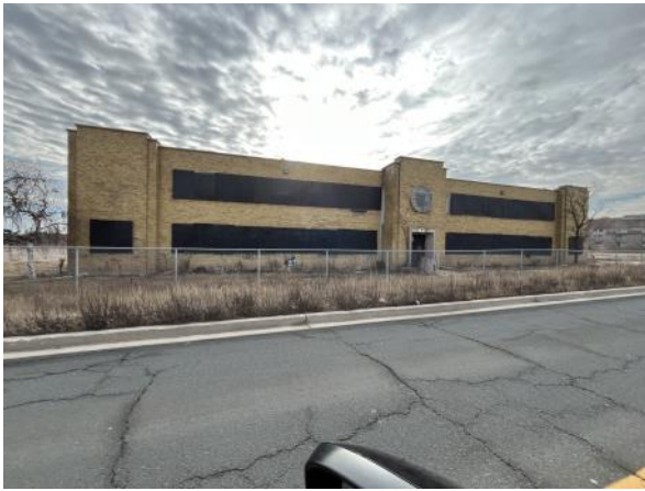
Photo 1: View of the boarded up Site heritage building (former offices) located on the north portion of the Site. Photograph taken facing southwest.
