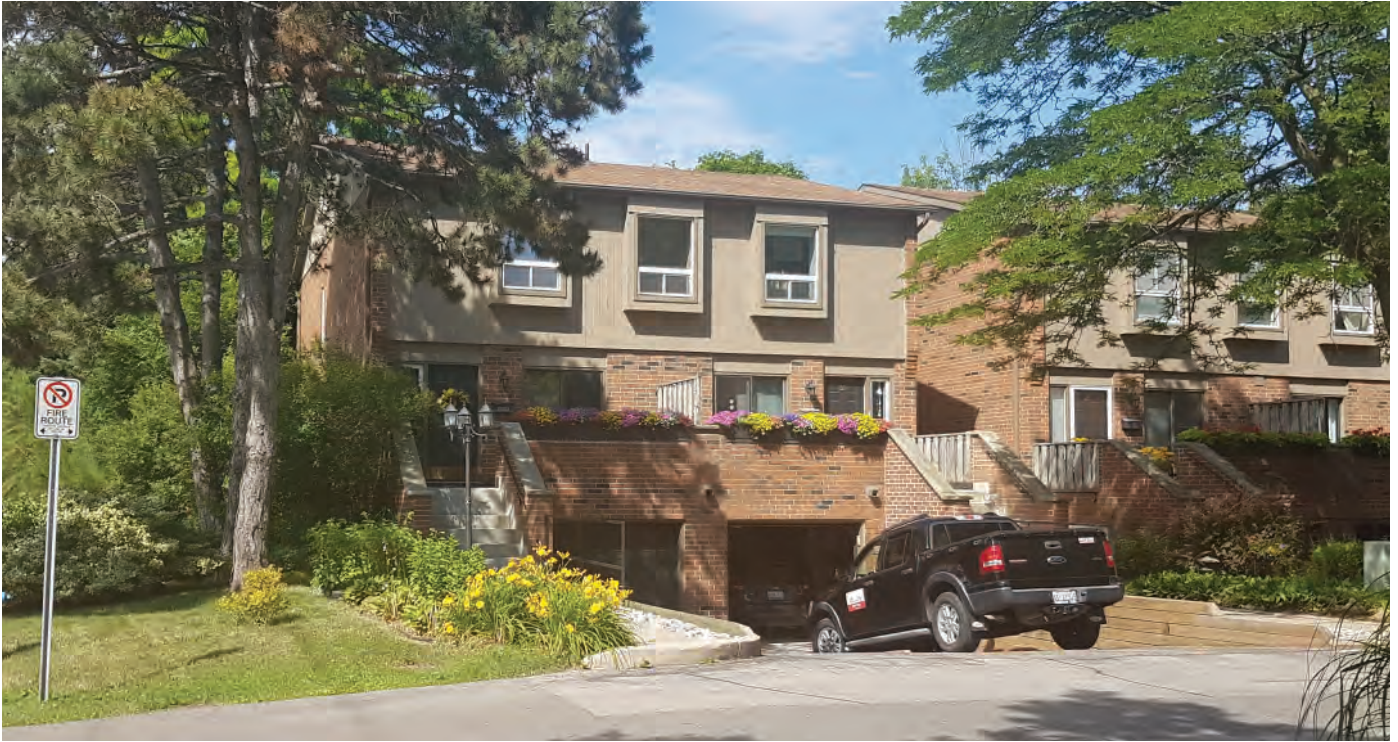
Figure 11: Entrance of semi-detached from Lakeshore Road West
