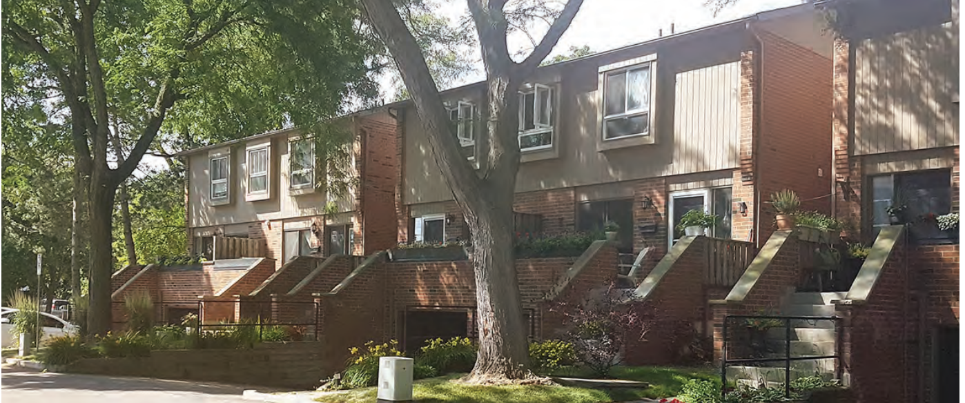
Figure 9: Existing semi-detached & townhouses at 3129 Lakeshore road West, southeast of the site
