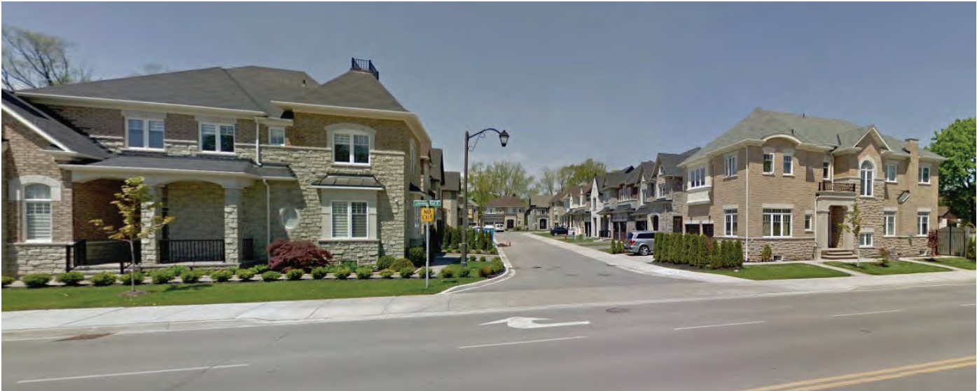
Figure 13: Entry to Waterview Commons with units facing Lakeshore Road West
