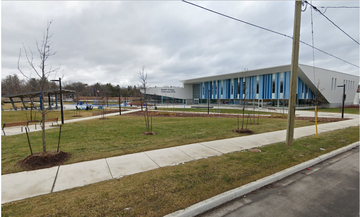
Photo 3: View of Oakville Trafalgar Community Centre and neighbourhood park from Reynolds Street facing east
