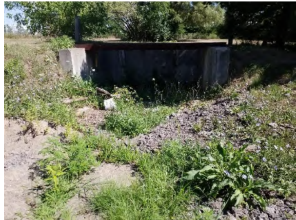
Plate 6: View of former foundation on the subject property, looking north.
