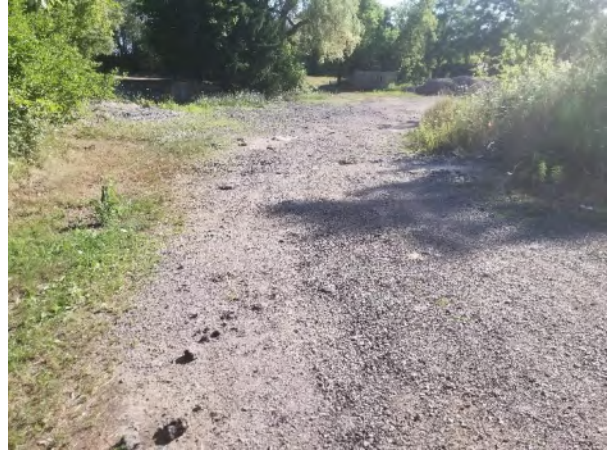
Plate 8: Gravel driveway in the western area of the property, looking east.
