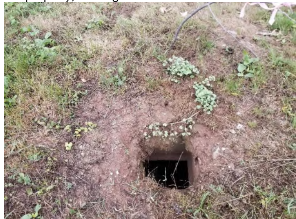
Plate 12: Subterranean drainage system south of the gravel driveway.
