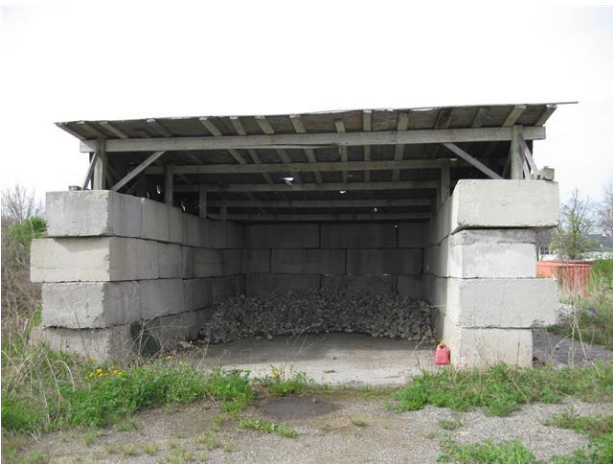
Photo 3: View of the concrete structure containing landscaping material.
