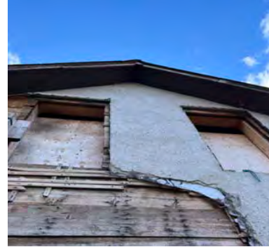
North elevation window units removed and openings boarded (ERA, 2023).
