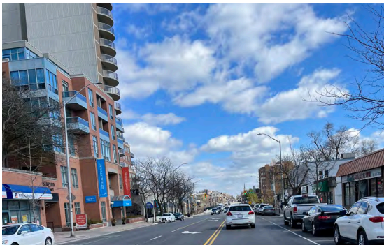
View east on Lakeshore Road West showing existing mid- and high rise residential buildings (ERA, 2023).
