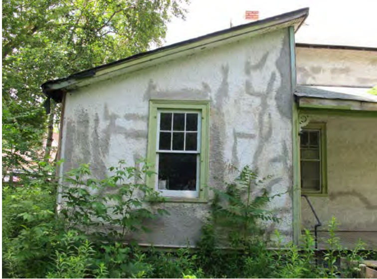
Rear portion of east elevation (ERA, 2011).
