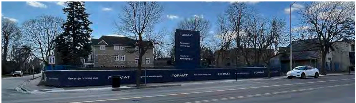
View of the Site along Lakeshore Road West (ERA, 2023).
