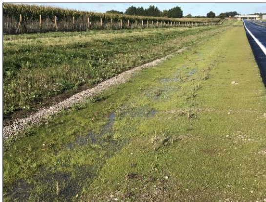
Example – Enhanced Roadside Swale (Source: TerrAffix)
