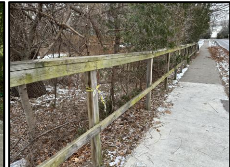
Wooden Railing Along South Side of Culvert Crossing
