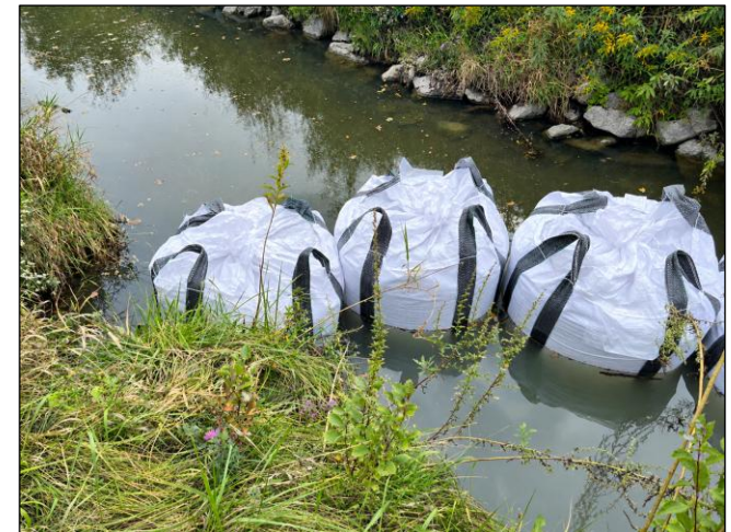
Example - Temporary Cofferd Dam
