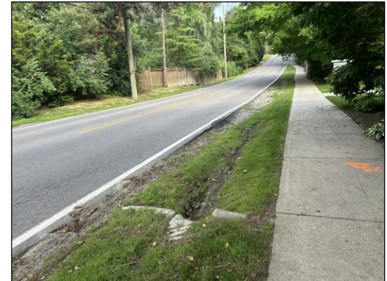
Existing CSP Culvert to be Retained
