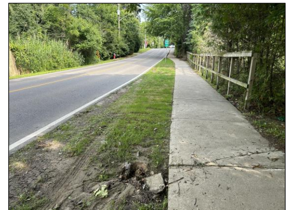
Existing Buried CSP Culvert to be Removed
