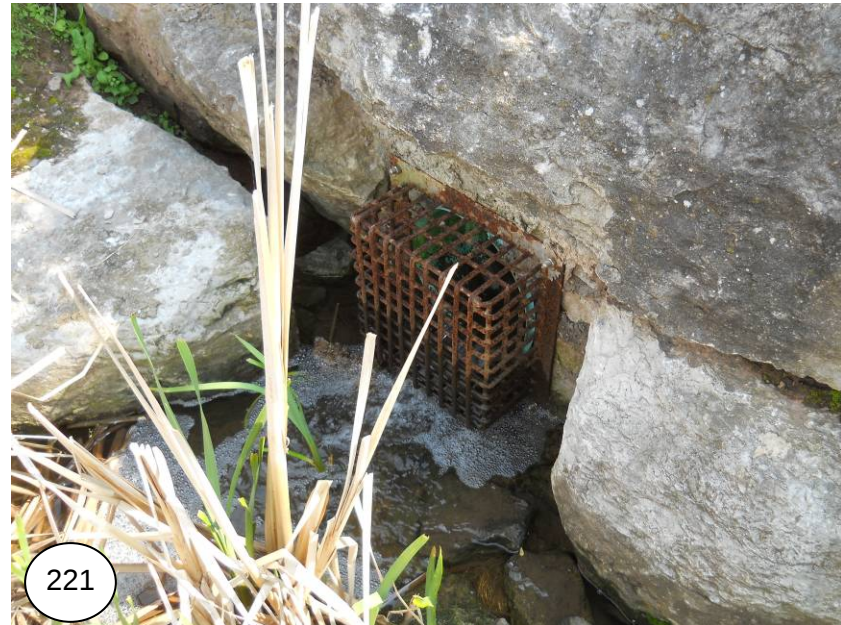
West Stormwater Management Pond outfall (detail)
