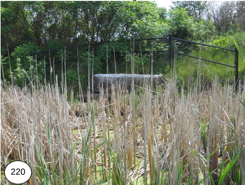
West Stormwater Management Pond outfall
