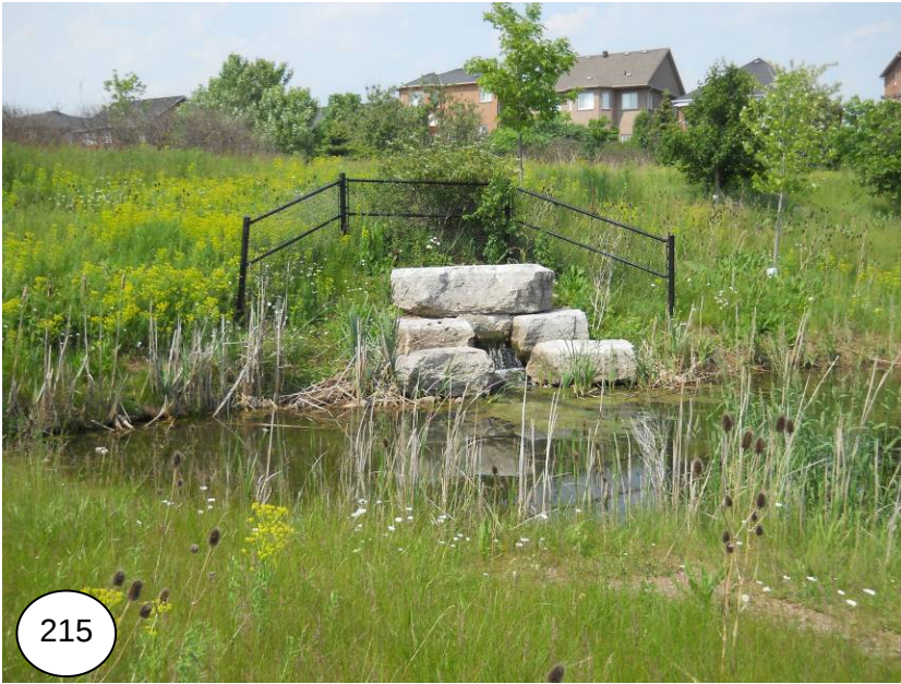
East Stormwater Management Pond outfall
