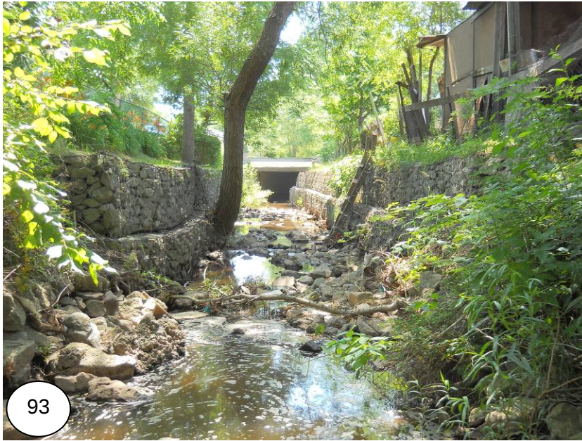
Looking downstream (Pinegrove Rd. crossing)
