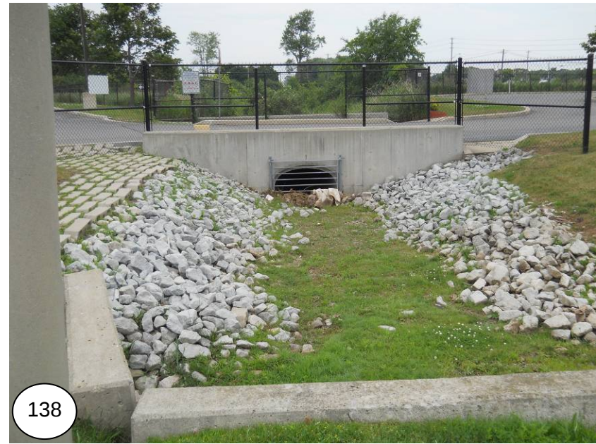
Redwood Square (Online Stormwater Management Pond inlet)
