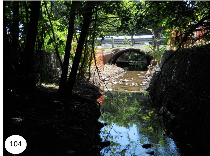
Looking downstream (Wildwood Dr. crossing)
