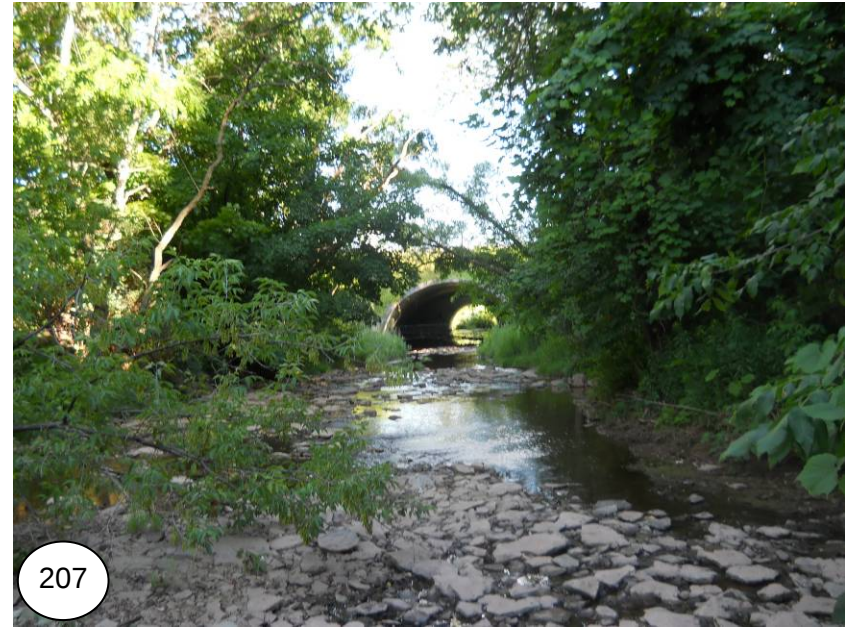
Looking downstream (North Service Rd. West crossing)
