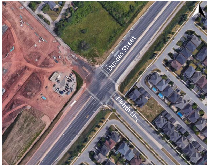
Figure 3: Intersection of Eighth Line at Dundas Street
