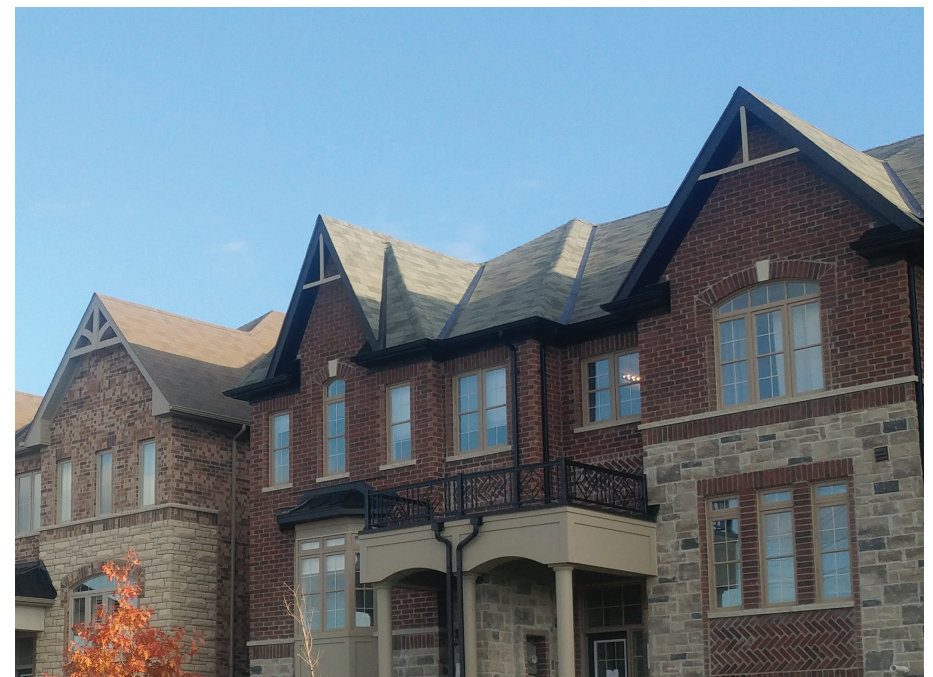
Traditional roof design
