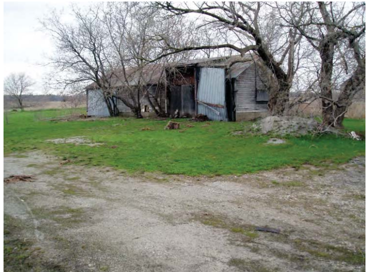
Plate 8 Area of Disturbance, View North
