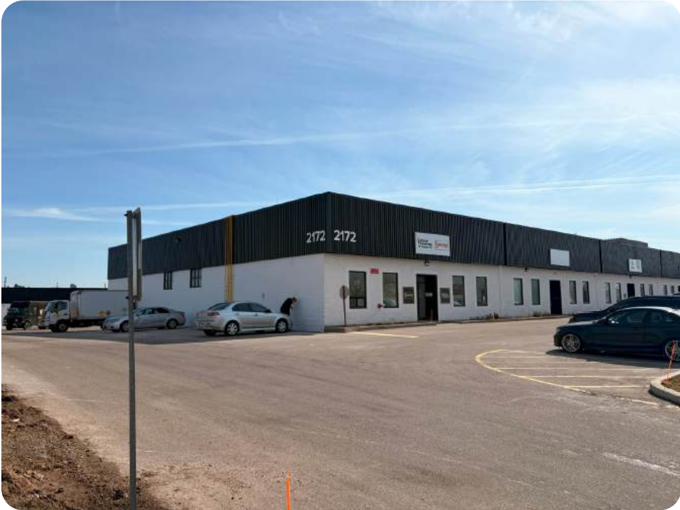
Subject Site, Looking Southwest
