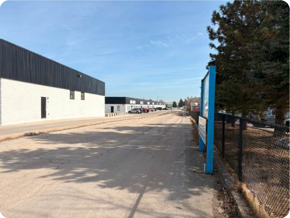
Subject Site, Looking Southwest
