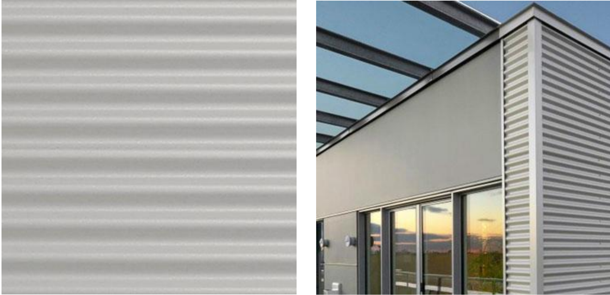
VICWEST 7/8" CORRUGATED PROFILE OR EQUIVALENT BASIS OF DESIGN COLOUR: FLUROPON 6724-SILVER
