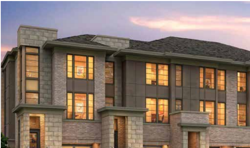
Contemporary roof design
