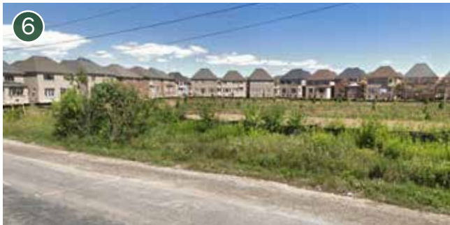
Existing single detached houses under construction backing onto NHS channel along east side of Sixth Line, south east of the Star Oak Development subject lands.
