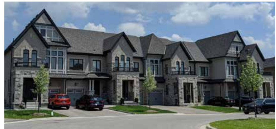
Fig. 6.3.3a - Built form within the neighbourhood will predominantly comprise single detached and townhouse residential, utilizing both contemporary and traditional architectural styles and themes.
