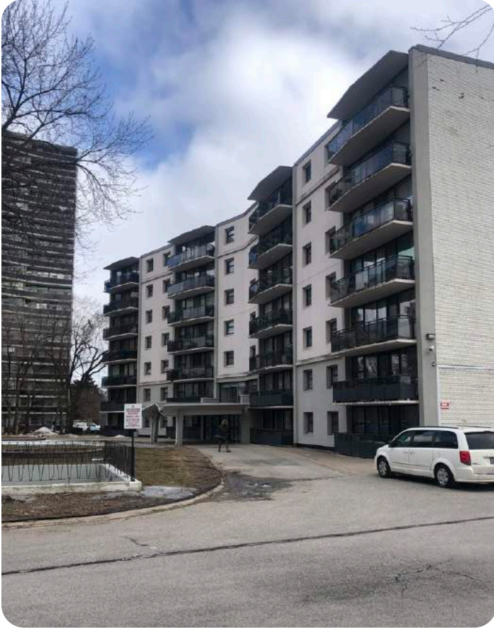
The existing 7-storey apartment building on the Subject Site, looking southeast
