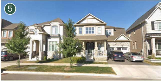
Existing single detached houses on Preserve Drive, south west of the Argo West Morrison Creek subject lands.
