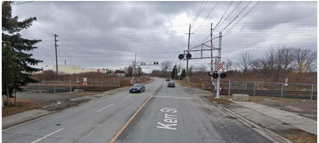
Existing condition of the at-grade railway crossing on Kerr Street
