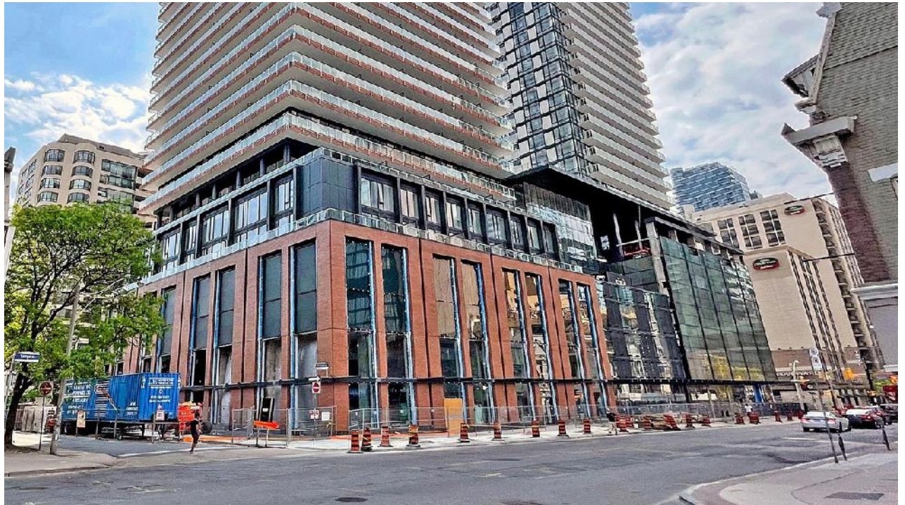
501 Yonge Street: Permeable facade with verticle architectural language shields the above ground parking structure
