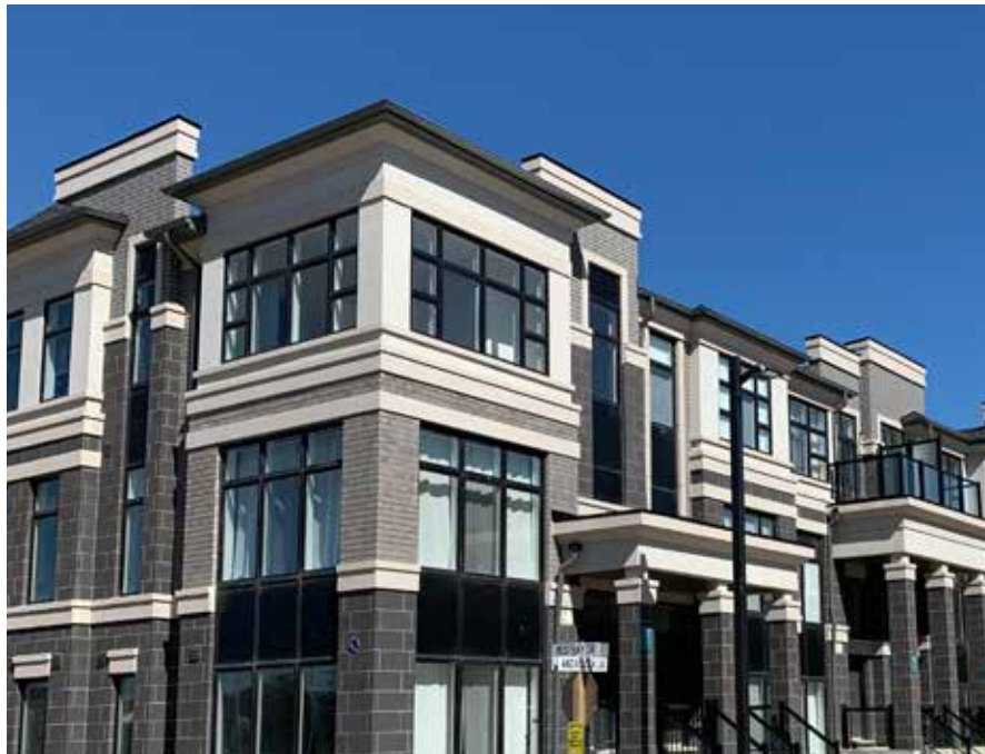
Contemporary roof design
