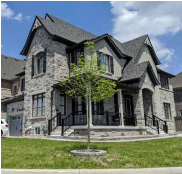
Fig. 4.9a - Example of a priority lot dwelling located at a corner that appropriately addresses both streets through architectural treatment (side-facing porch, wall articulation, windows, etc.)
