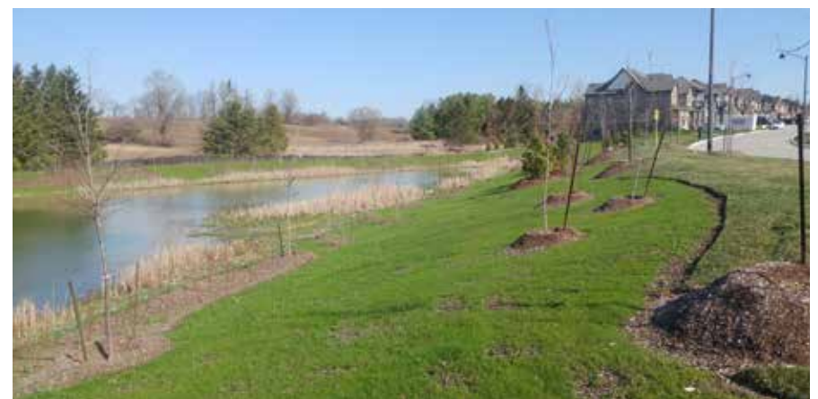
Fig. 2.2.3 - Image examples of a SWM pond facility adjacent to existing natural heritage features and residential use.
