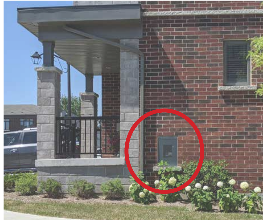
Fig. 4.7 - Utilities should be discreetly located, integrated into the architecture or screened from public view
