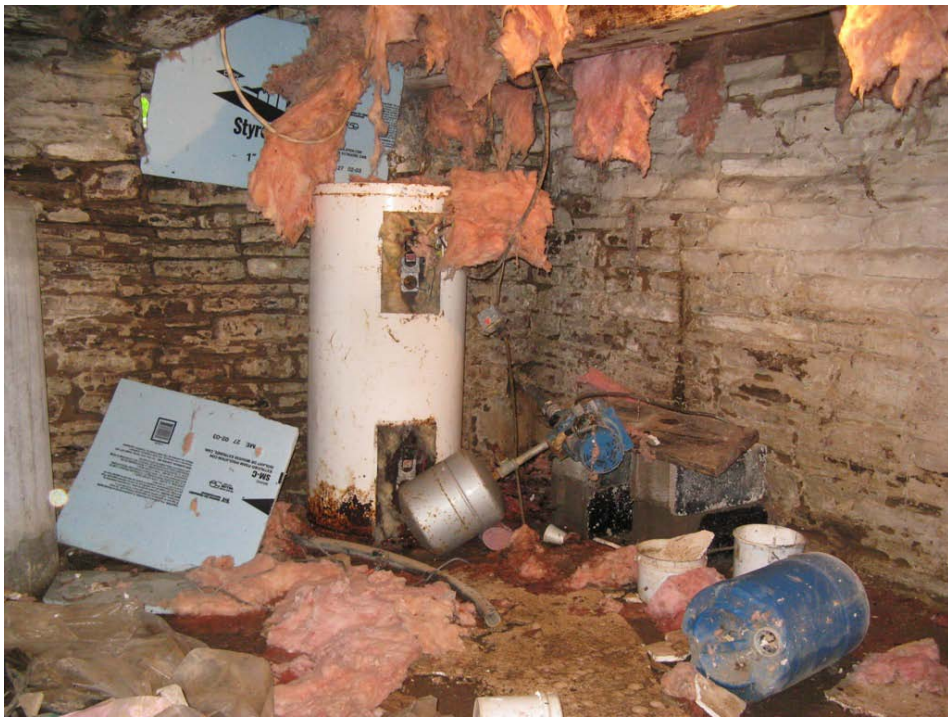
Photograph 17: View of the basement of the house.
