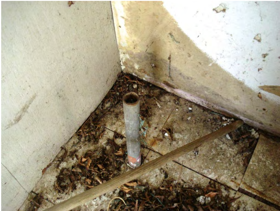
Photograph 16: Pipe observed in the mudroom of the house.
