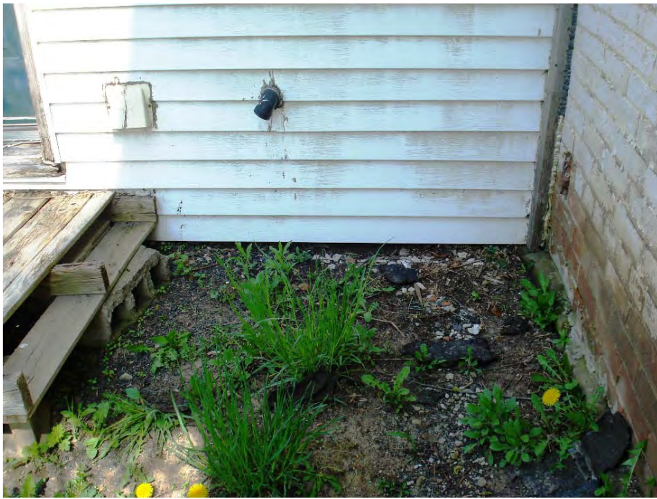
Photograph 19: Pipe observed on the southern wall of the house.
