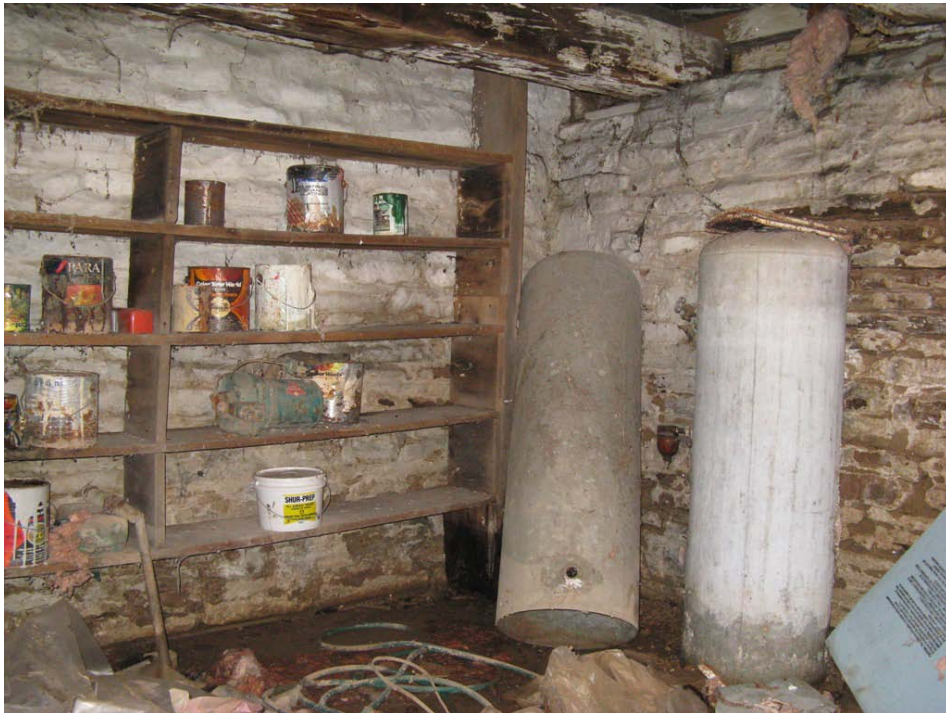
Photograph 18: Paint cans and storage observed in the basement of the house.
