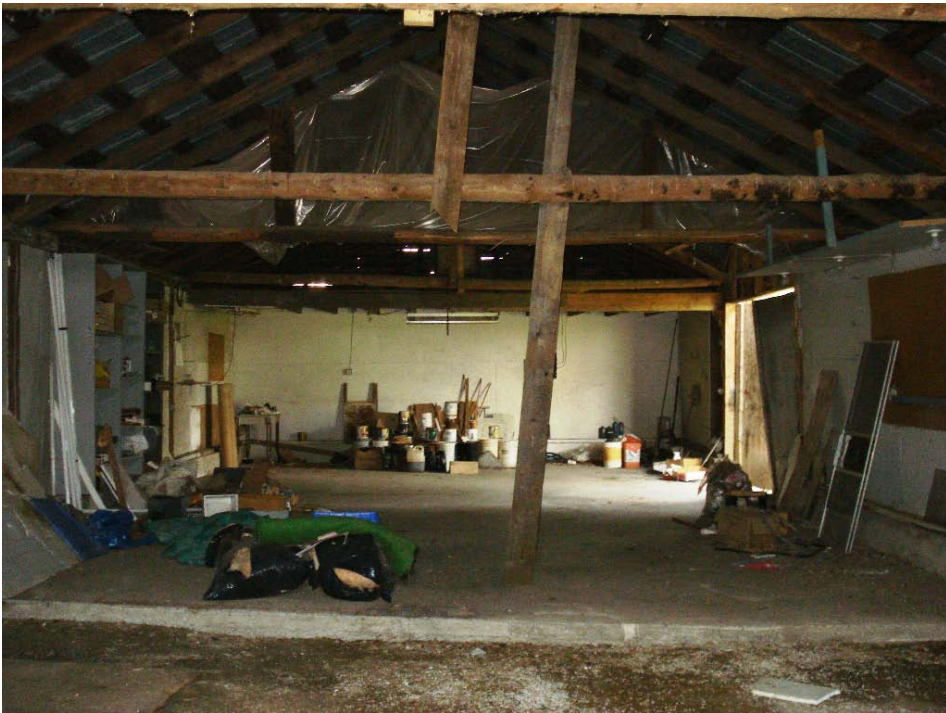
Photograph 14: General view of storage within the large shed.
