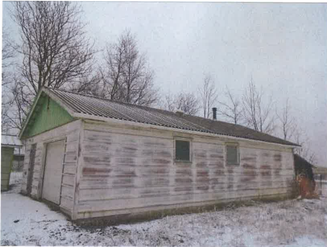
General view of the garage at 2460 Old Bronte Road (facing southwest)
