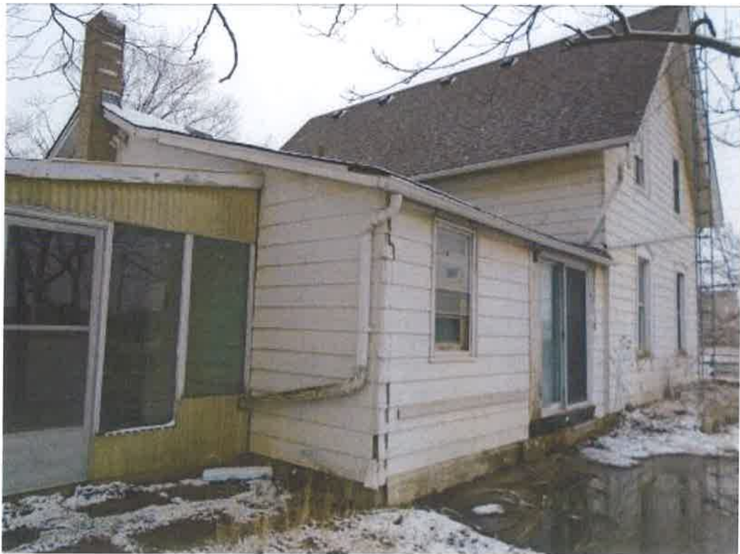
View of the south façade of 2460 Old Bronte Road (facing northeast)
