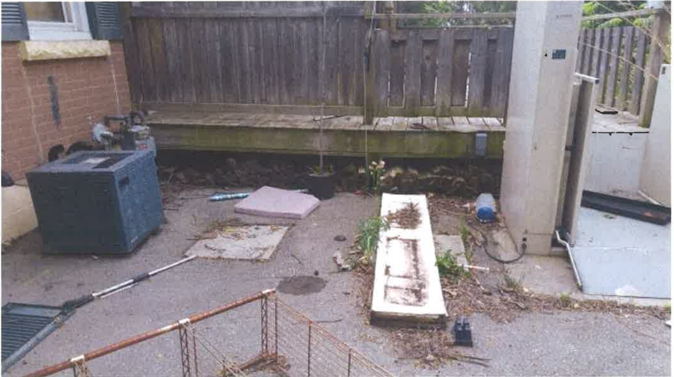
View of an electrical elevator at 2454 Old Bronte Road (facing south)
