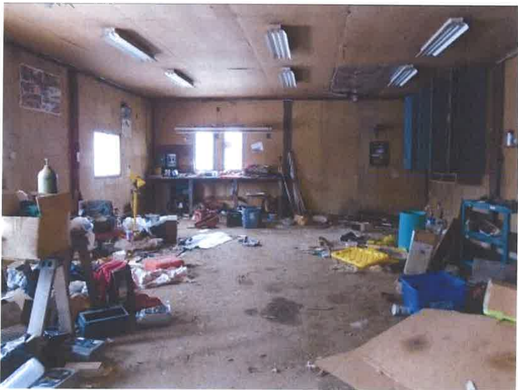
General view of a barn at 2444 Old Bronte Road (facing south)
