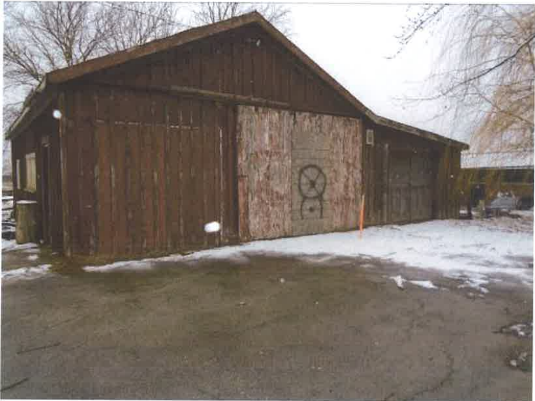
General view of a barn at 2444 Old Bronte Road (facing southwest)
