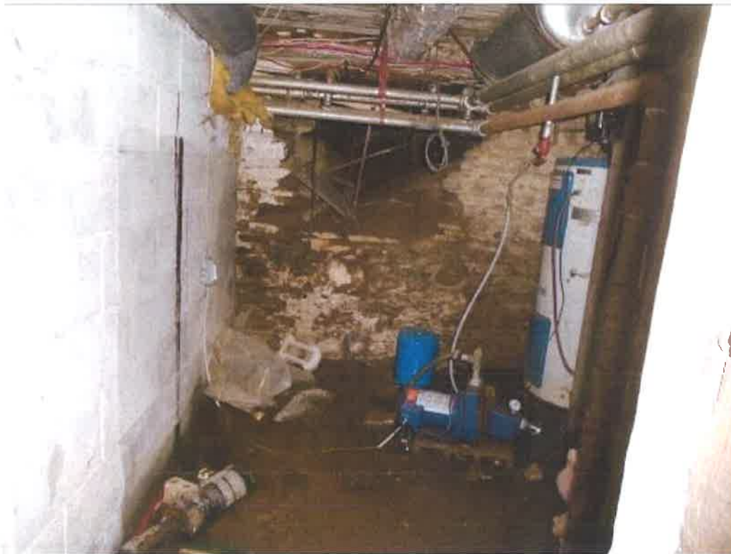
General view of the basement of 2460 Bronte Road (facing south)
