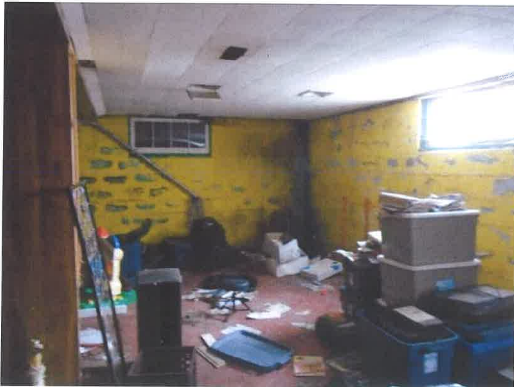
View of the basement at 2444 Old Bronte Road (facing north)
