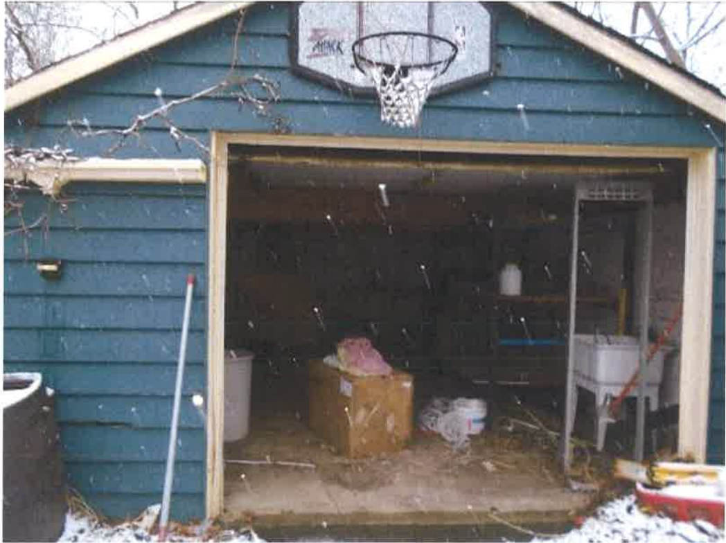
General view of a garage at 2454 Old Bronte Road (facing west)
