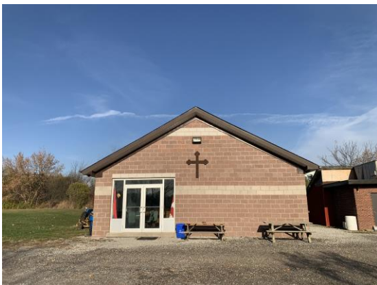
Picture 17: View of the eastern elevation of Site Building C, facing east.
