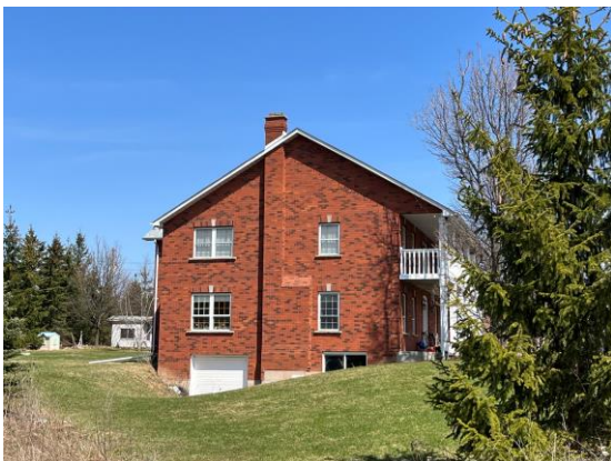
Picture 5: View of the western elevation of Site Building A, facing east.
