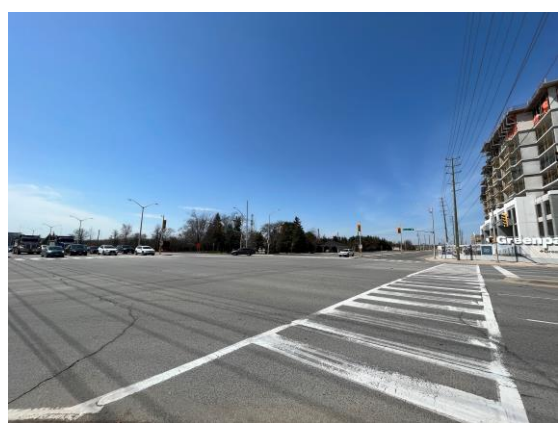
Picture 36: View of the intersection of Neyagawa Blvd and Dundas St W, facing north.
