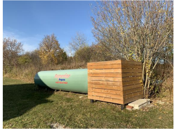
Picture 20: View of the propane tank on the northern portion of the Property, facing northeast.
