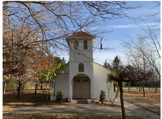
Picture 22: View of Site Building E, facing south.
