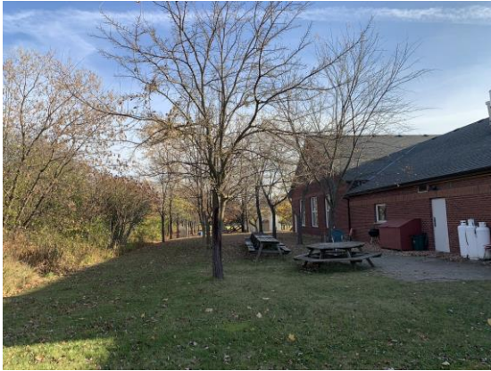
Picture 19: View of the southern elevation of Site Building D, facing south.
