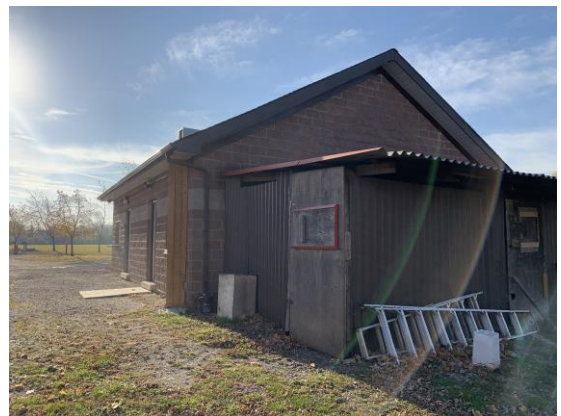
Picture 18: View of Site Building C and Shed 3, facing northwest.
