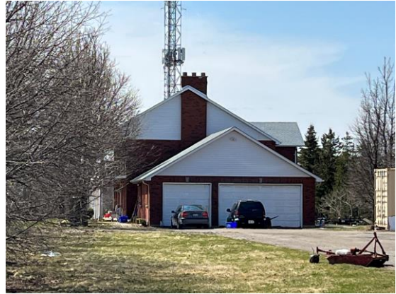
Picture 2: View of the eastern elevation of Site Building A, facing west.
