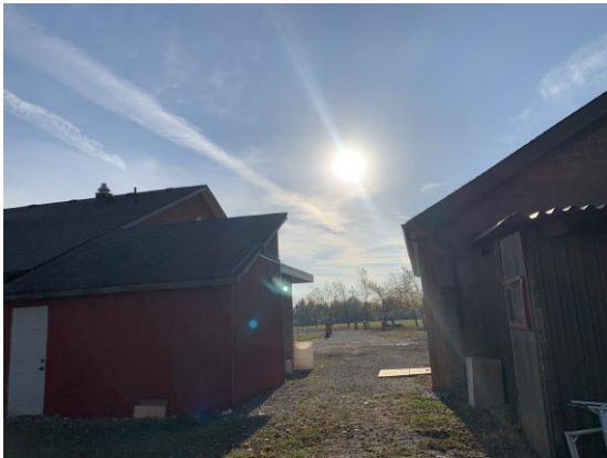
Picture 21: View of Site Buildings C and D, facing west.
