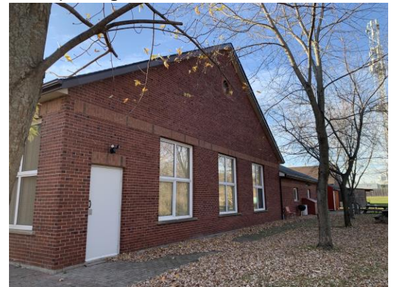
Picture 16: View of the eastern elevation of Site Building D, facing northwest.
