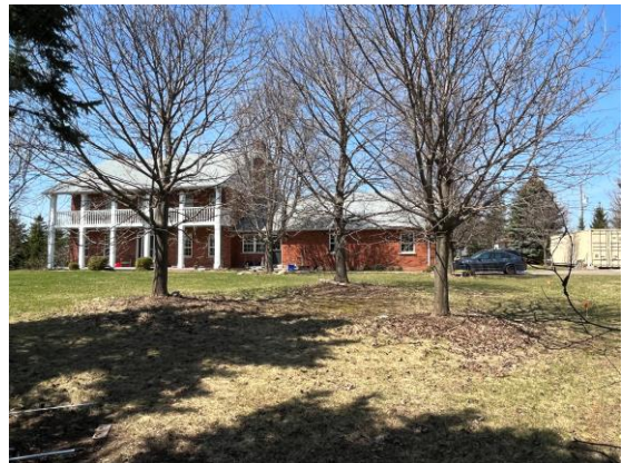
Picture 4: View of the southern elevation of Site Building A, facing north.
