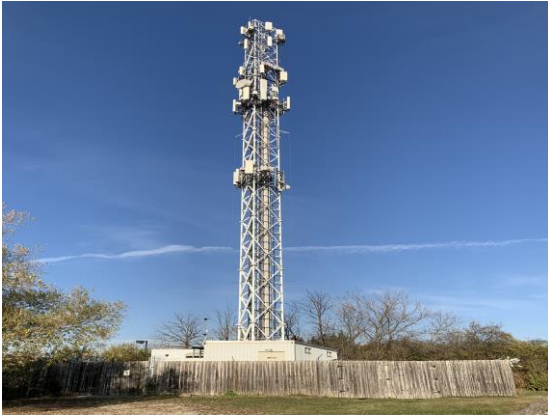
Picture 25: View of the Telus telecommunication tower along the north Property boundary, facing east.
