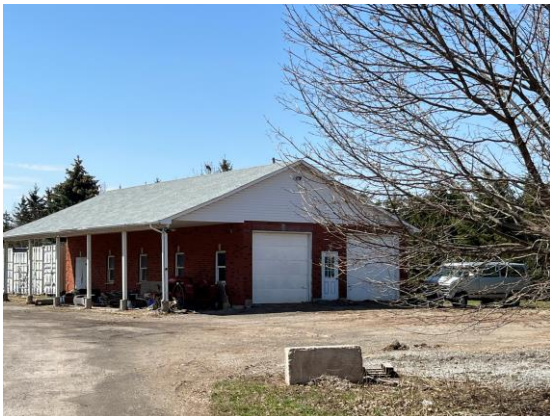
Picture 3: View of the eastern elevation of Site Building B, facing west.
