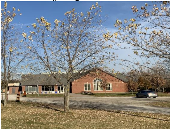
Picture 15: View of the western elevation of Site Building D, facing east.
