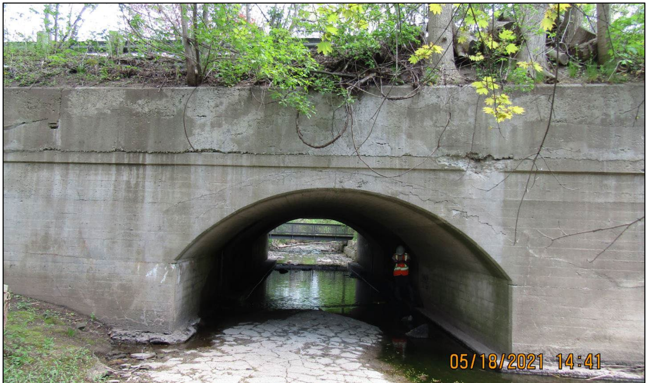
Figure 1-2: Photograph showing arch structure of McCraney Creek Bridge
