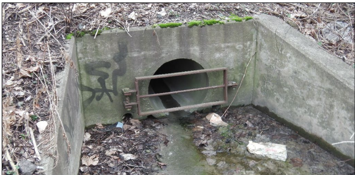
Figure 3-8: Photograph of Storm Outfall
