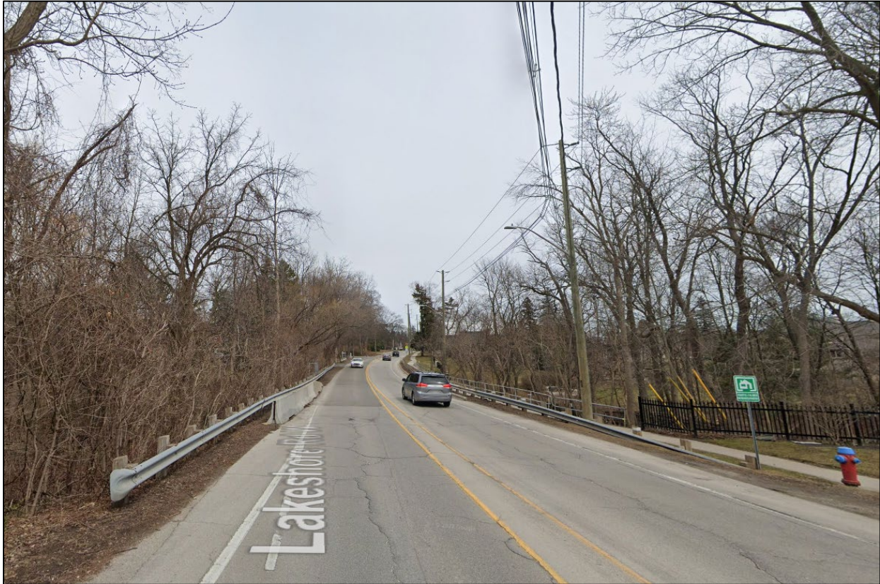
Figure 3-9: Google Streetview Showing Hydro Poles on the South Side of Lakeshore Road West
