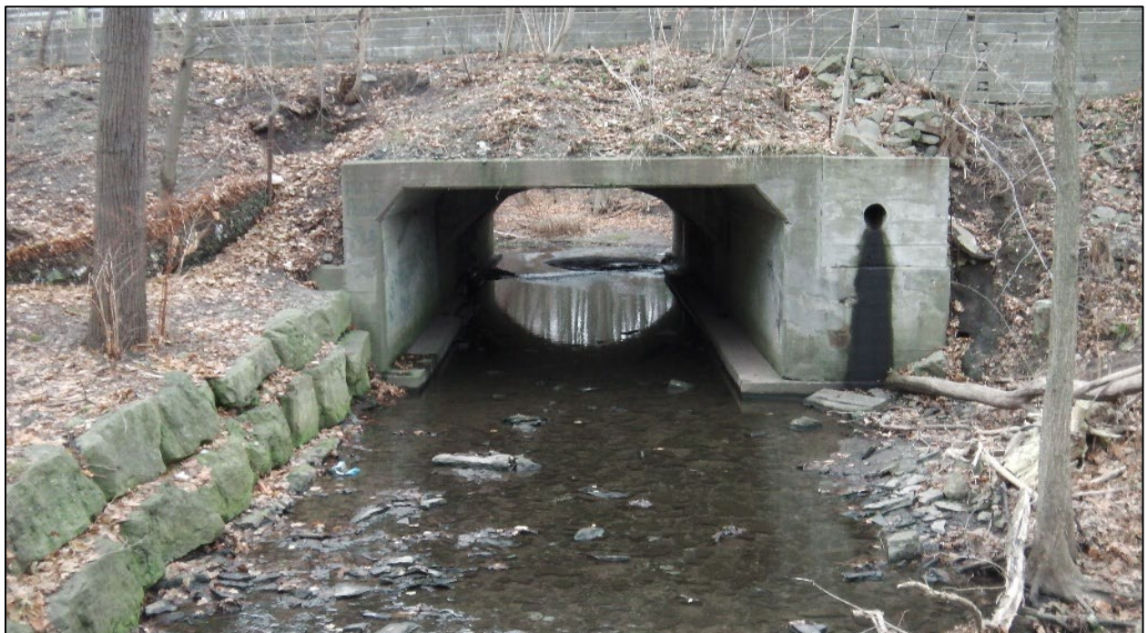
Figure 1-3: Photograph showing box culvert extension of McCraney Creek Bridge
