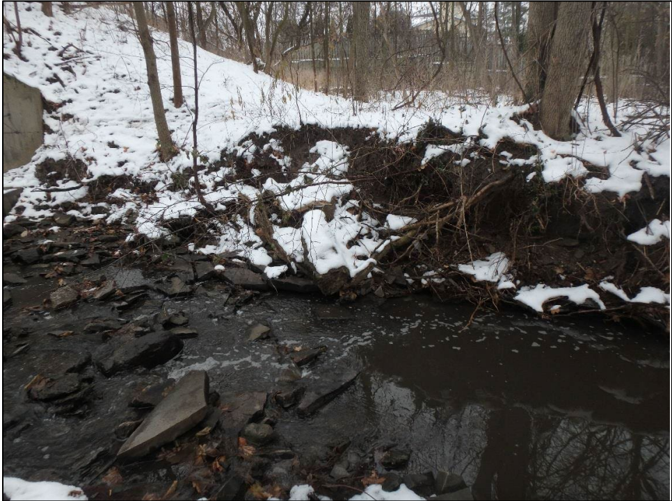
Figure 3-18: Erosion along East Bank of McCraney Creek
