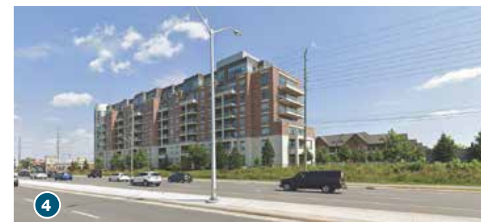
8-storey apartment building at Dundas Street East and Prince Michael Dr
