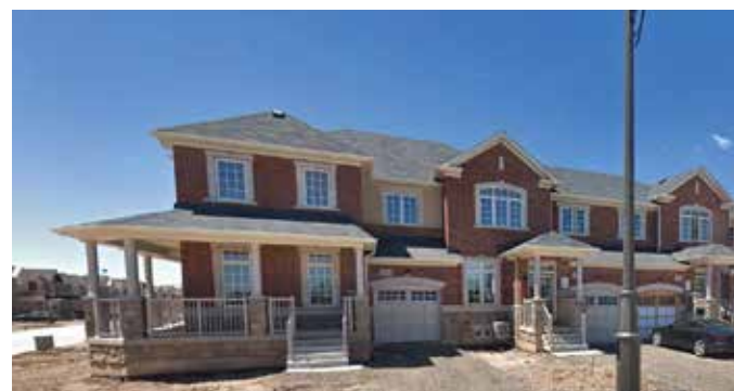
Townhouse units on Threshing Mill Blvd.
