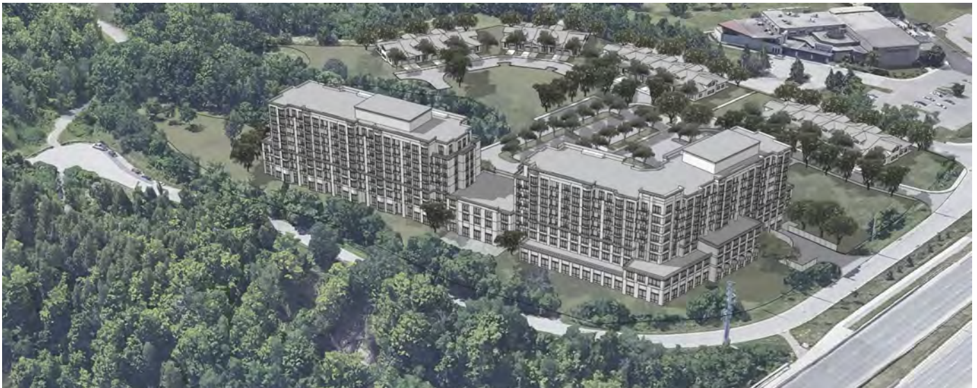
As illustrated, the eight-storey seniors residence has been designed with stepbacks above the podium base. A three-storey podium connects the two towers, which breaks up the overall building mass. The building has been oriented towards surrounding roads including Fourth Line and Dundas Street West and is oriented to provide views of Sixteen Mile Creek.
