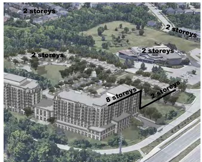
The above graphic illustrates how building heights transition from 8 storeys to 2 storeys with the lower building heights located in proximity to the St. Volodymyr Cultural Centre and existing low rise residential communities.
