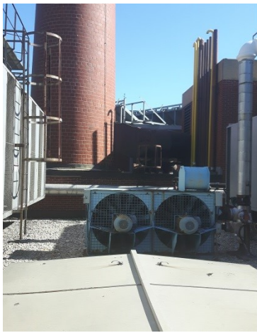
Photo 15: View of smoke stack / chimney located on the northwest portion of the former hospital building.
