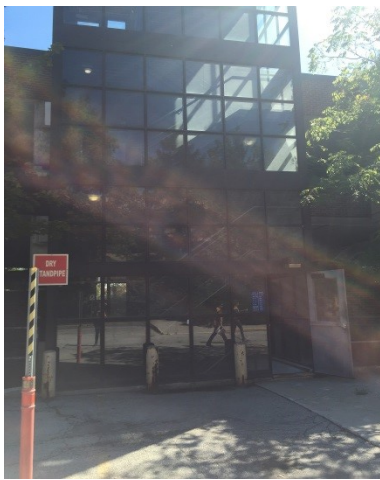
Photo 9: View of the west side of the parking garage (facing east).
