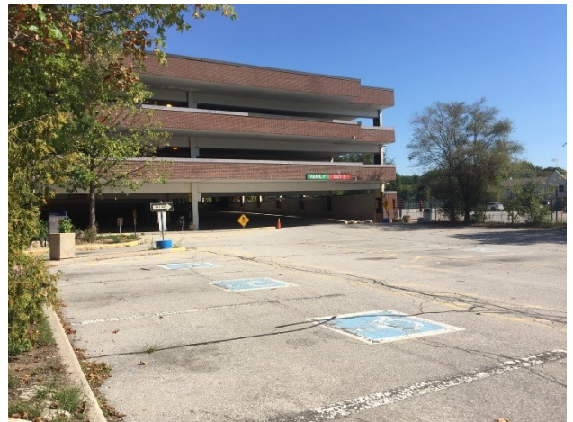
Photo 18: View of the north side of the parking garage and parking area (facing south).
