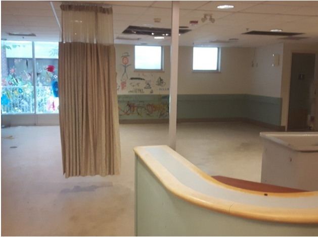
Photo 1: View of the interior of the former hospital building.
