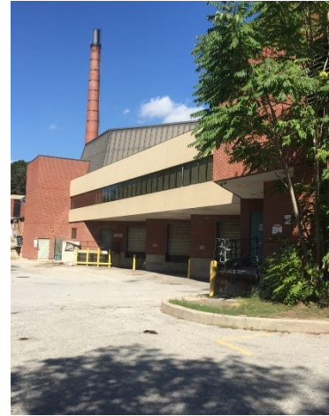
Photo 8: View of the west portion of the former hospital building showing the smoke stack/chimney (facing NE).
