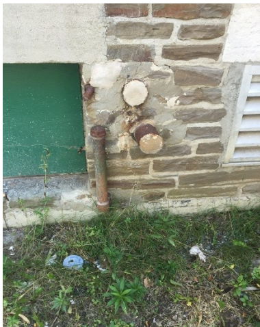
Photo 11: View of the fill and vent pipes observed on the former school building (east side of building).
